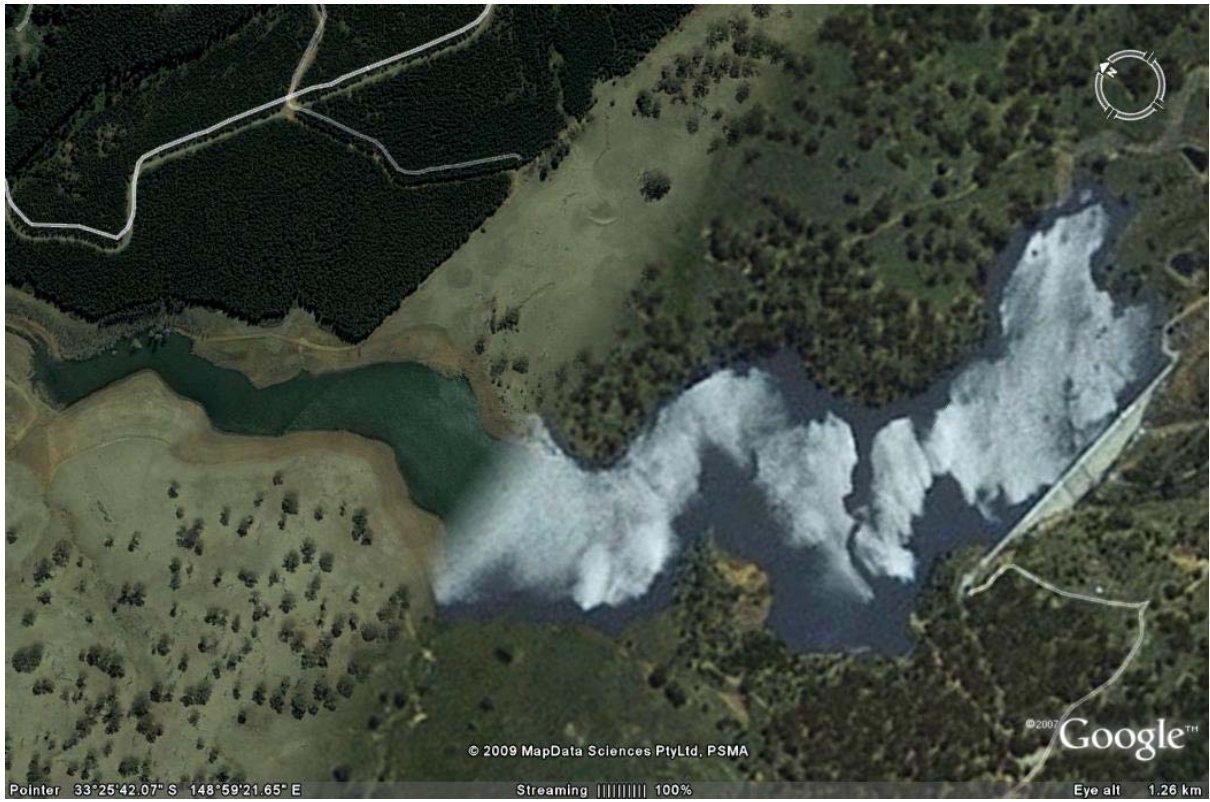
Google Earth View of Rodd's Creek Dam
