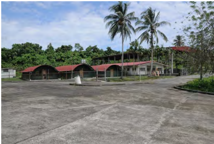
Figure 7 Existing Infrastructure at Fisheries (SKM, 2013)
