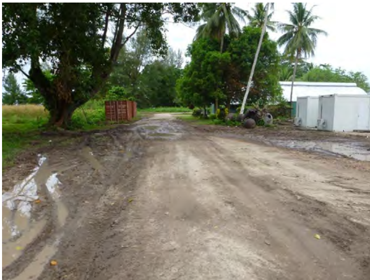
Figure 5 Hardstand Site 1 (SKM, 2013)
