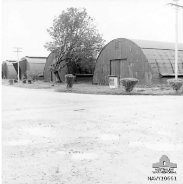
Figure 18: Nissen (or Quonset) Huts at Lombrum Point c 1950 (Source: Australian War Memorial)
