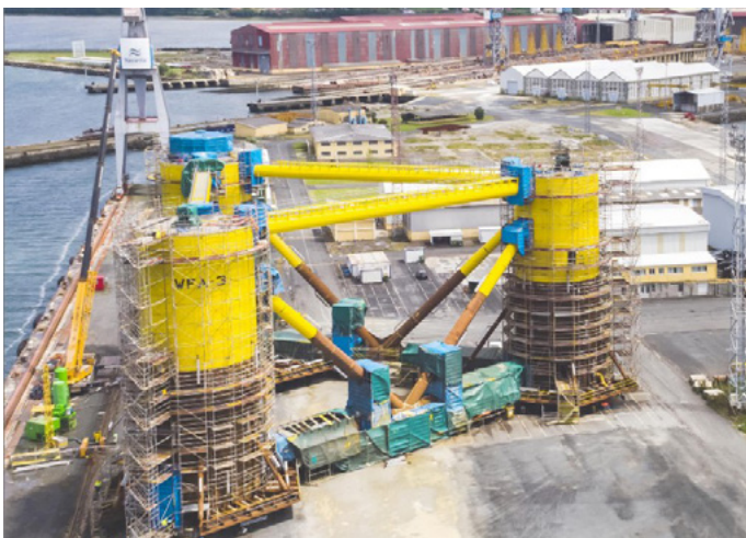
Figure 9: Semi-submersible foundation under construction at port. (Wind Europe, 2020) (Photo: Navantia)
