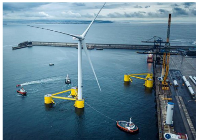
Figure 10: Semi-submersible foundation being towed to location. (Wind Europe, 2020) (Artist: Dock90)
