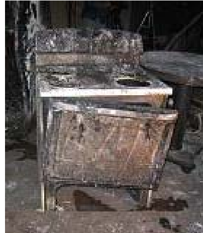
Stove (post fire)
