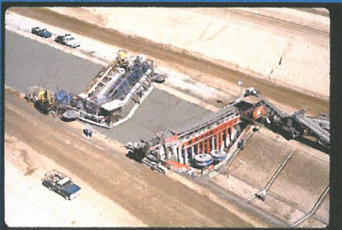
Paving canal liner
