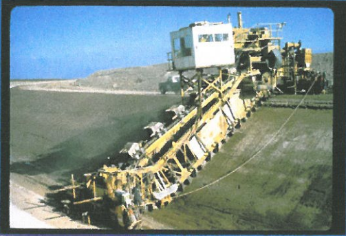
Paving The Aqueduct
