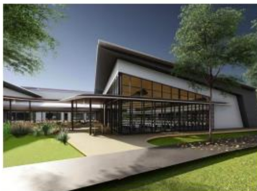
External view of messing facility
