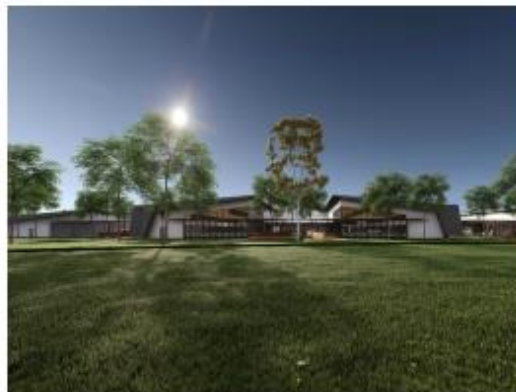
External view of mess facility
