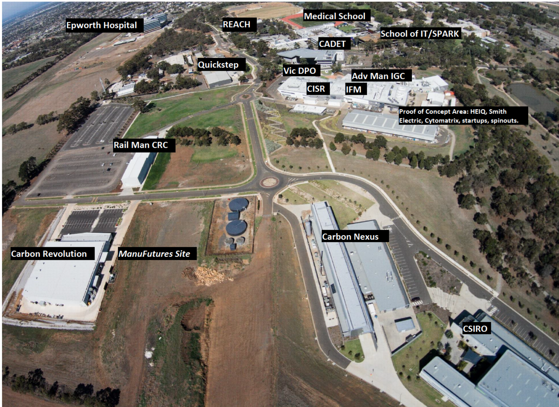
Aerial view of the Geelong Innovation Precinct February 2016
