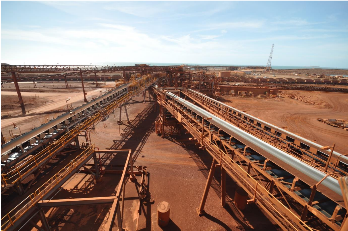
Figure 8 The tracked components can be monitored all the way to installation in connection with the digital model
