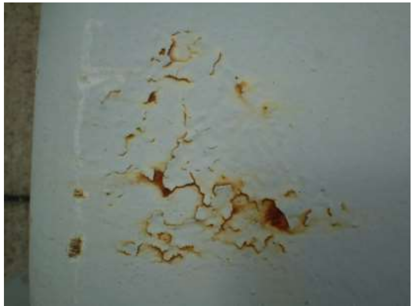
Photo 8 Poor paint finish against a specification of 75um inorganic zinc silicate, 125um Epoxy and 75um urethane
