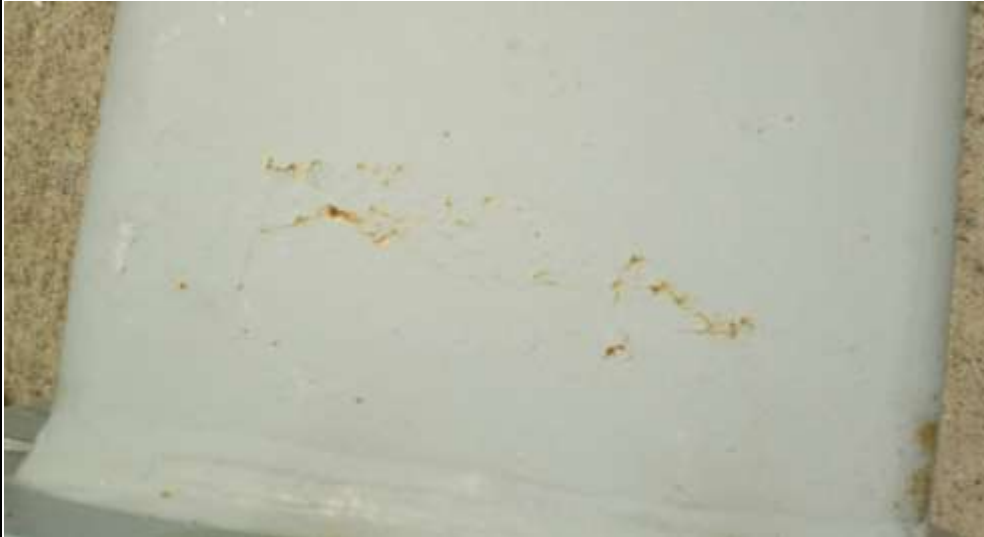
Photo 8 Poor paint finish against a specification of 75um inorganic zinc silicate, 125um Epoxy and 75um urethane
