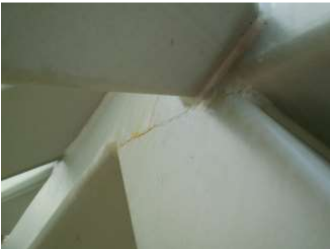
Photos 11- 14 Cracking across the section
