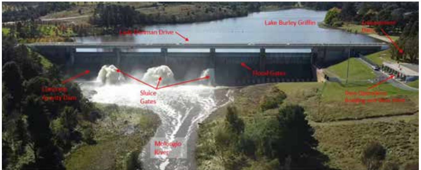
Figure 2.3 General arrangement of Dam
