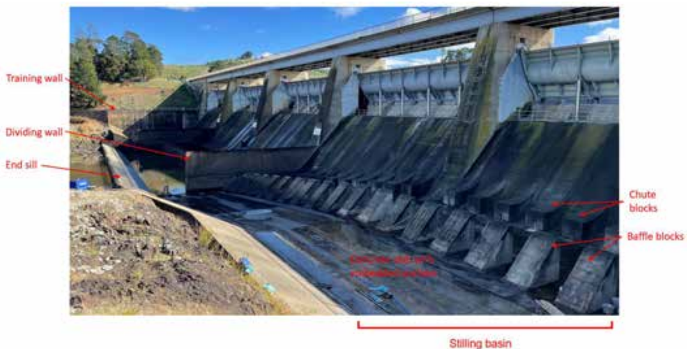
Figure 2.4 General layout of Scrivener Dam dissipator
