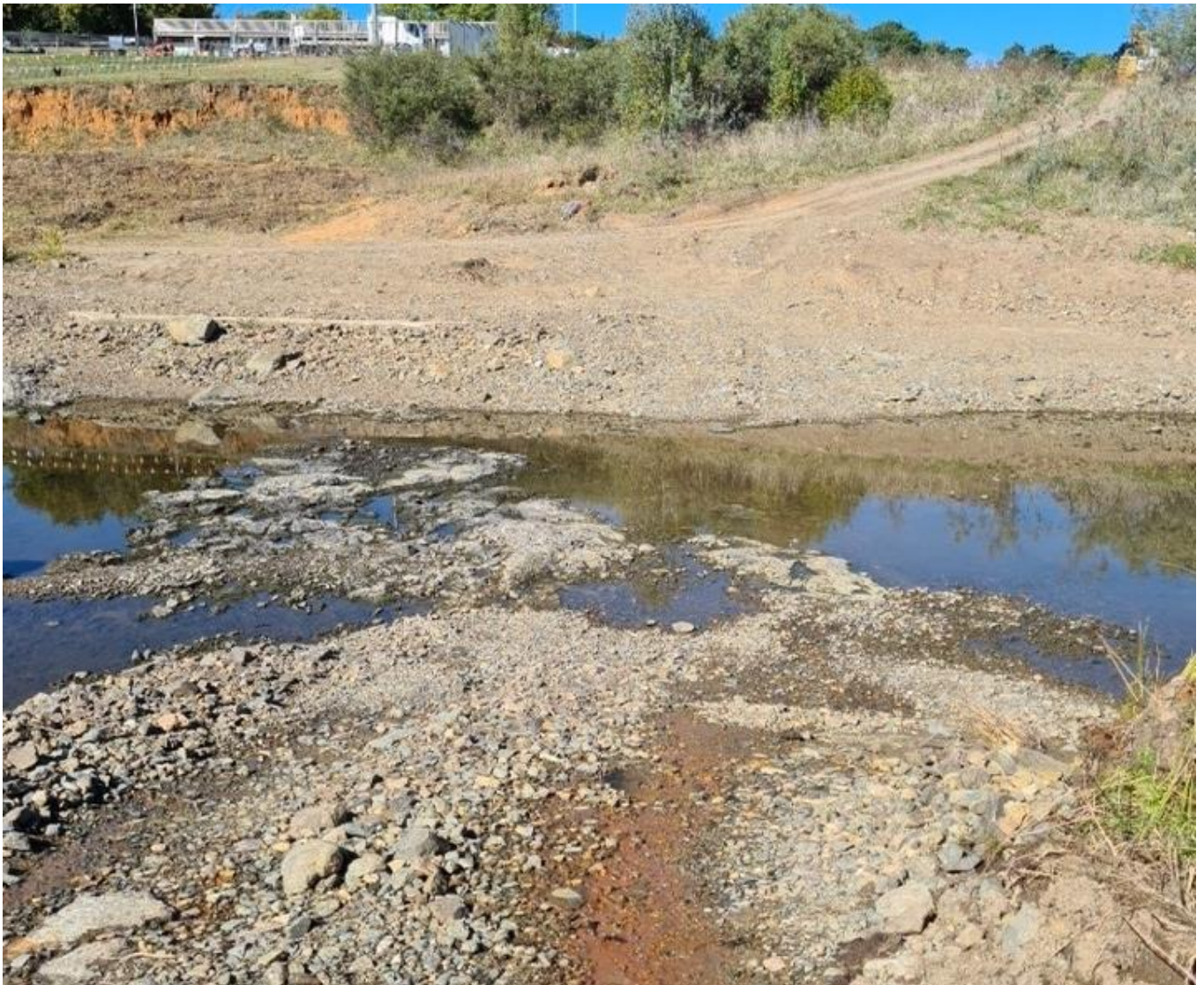
Figure 5.5 River crossing and temporary track leading up towards main office
