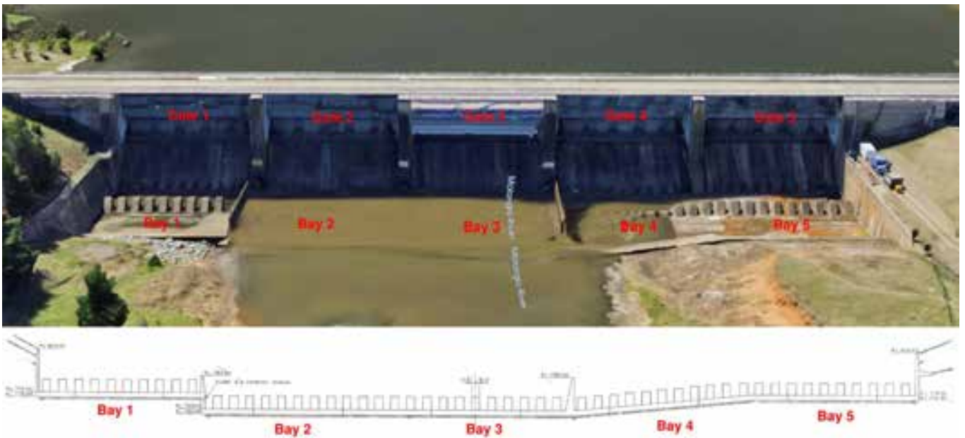
Figure 2.8 Numbering of bays and gates within Scrivener Dam
