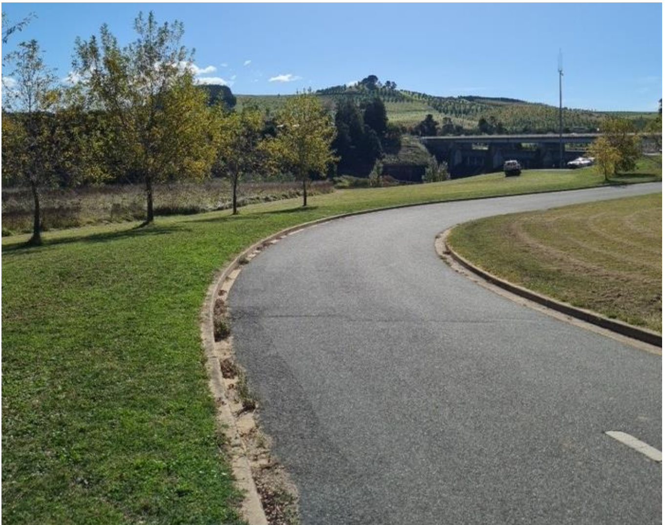
Figure 5.15 View from main entry to Scrivener Dam
