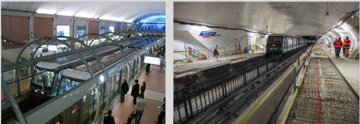
Figure 1: automated metro lines in Paris, France. Left: line 14, first high-capacity fully automated metro line released in the world. Right: on-going implementation of Platform Screen Doors on line 4, converted to automation without interrupting operation. Source: RATP
