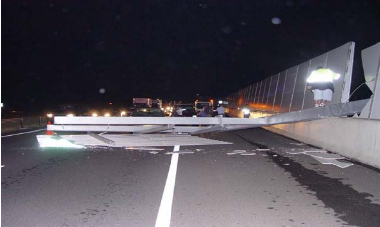
Photo 1 Bolts failure
