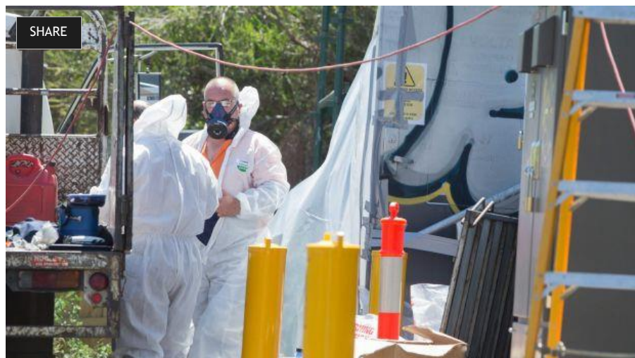
Workers prepare to remove asbestos from the substation in Thornbury. Photo: Simon Schluter
