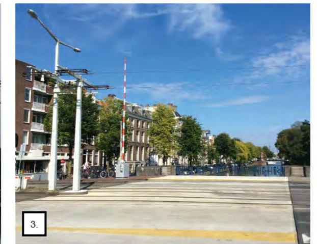
3. DOUBLE BASCULE BRIDGE HORTUSBRUG, AMSTERDAM
