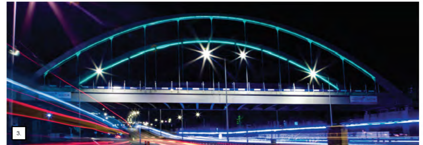
1. TRAMLINE TRUSS BRIDGE, THE HAGUE 2. 3. TRUSS BRIDGES, NOTTINGHAM TRAMLINE
