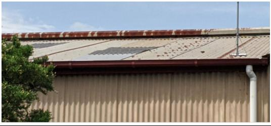
4. External cladding damage and deterioration that could not be replaced. This makes the shed vulnerable to break ins.
