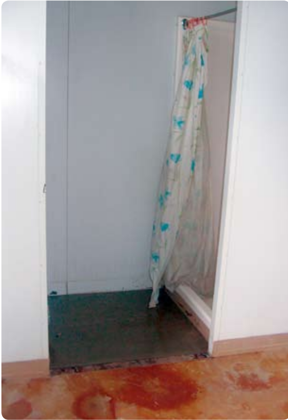
..... Shower block, Phosphate Hill immigration detention facility
