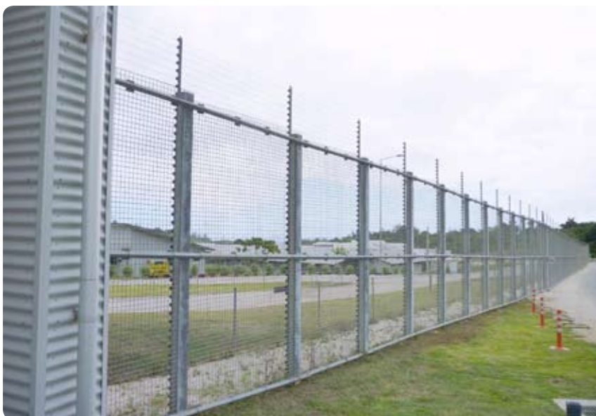
..... External fence, Christmas Island IDC
