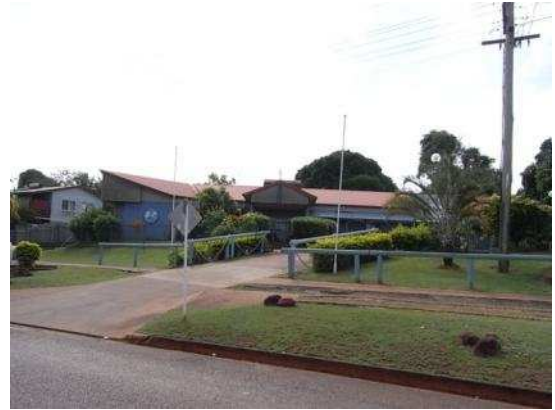
NPA Regional Council Office Bamaga
