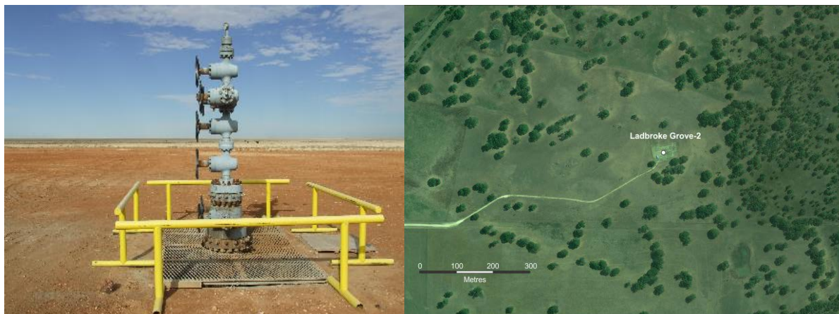
Figure 11: Wellhead in Cooper Basin (Strzelecki Desert) after stimulation and testing (left) and production wellsite in Otway Basin (Ladbroke Grove 2) rehabilitated to reduced lease area.
