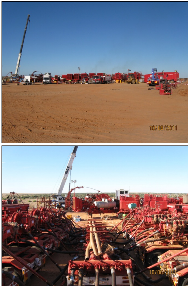
Figure 8. Fracture stimulation operations at Beach's Holdfast-1 well (Cooper Basin) in 2011
