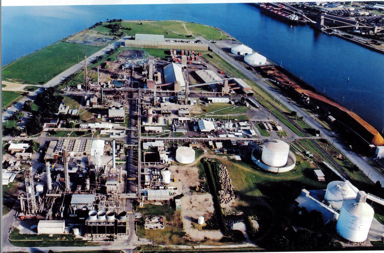
Orica's Kooragang Island plant.
