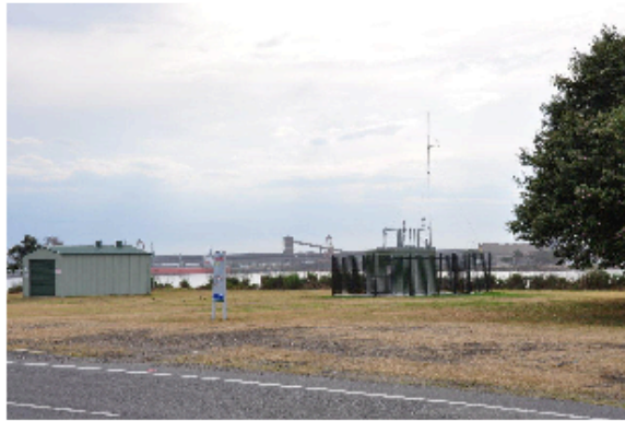
Orica Air Quality Monitoring Station Stockton
