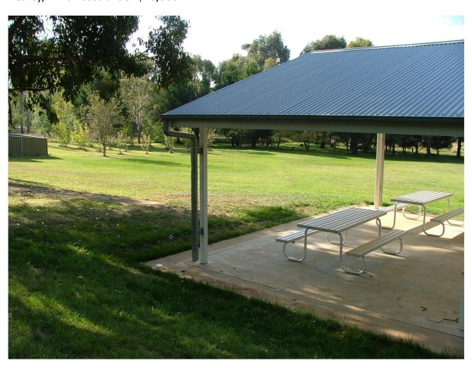
The roof drains do not connect to water tanks which is a pity as any rain will be wasted.
