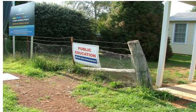
The Main Entrance to the school, showing the construction of the fence and the disconnected strainer. Approximately 80 meters of fence is in the same or worse condition, and should be replaced. Vehicle and pedestrian gates are needed to facilitate entry to the playground area for emergency vehicles - ambulance or fire brigade for example. Emergency services would have to knock down a portion of the rickety fence to gain access to the playground. A gate can't be attached to that post!
