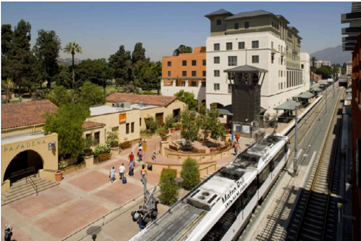
Figure 57: Metro Rail, Del Mar Station, Pasadena. Photo: Stefanos Polyzoides
