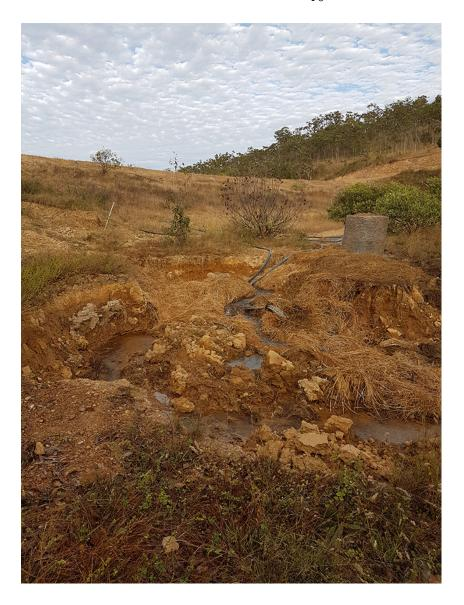
Environment Department staff drain a 1000 megalitre dam with a syphon hose on Springvale causing deep erosion and many hundreds of tonnes of sediment to flow into the adjacent East Normanby River and onto the Great Barrier Reef
