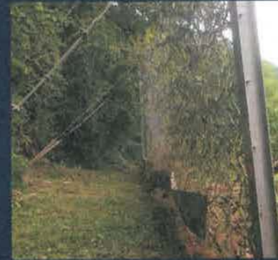
The rockfall fences are past their design life and need to be replaced.
