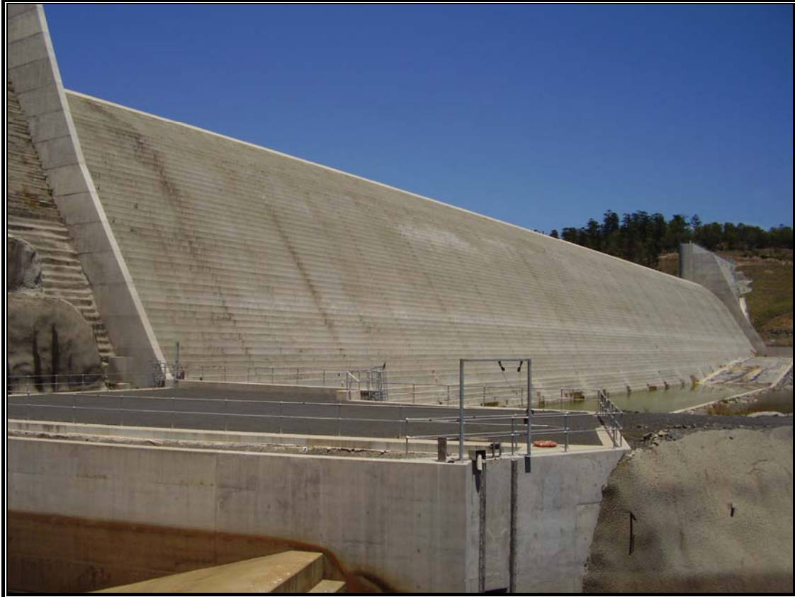
Image taken at the dam indicating the stepped design and shallow plunge pool .
