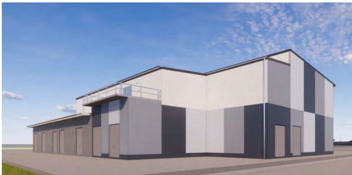
Shore Power Station 2
