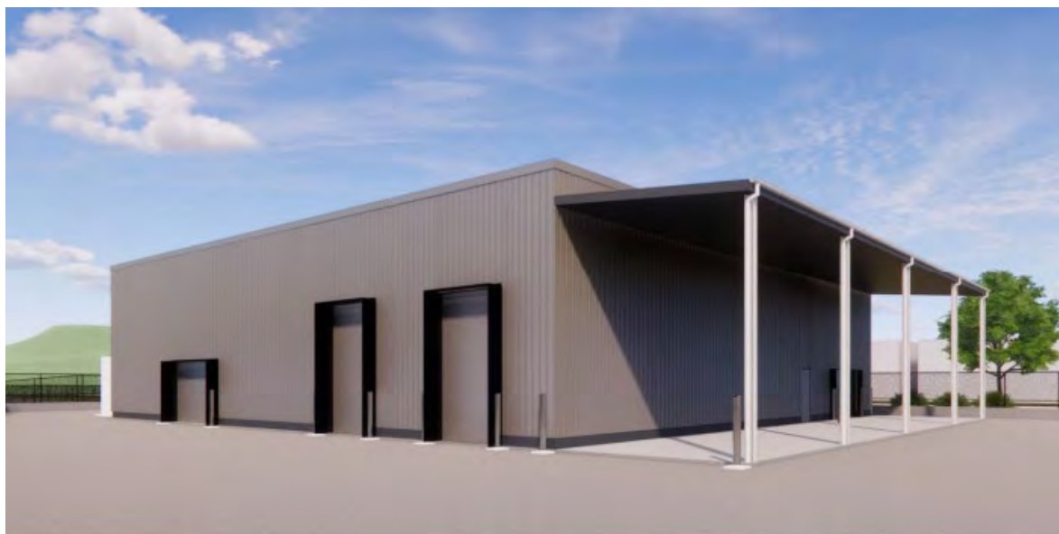
Pure Water Processing Plant
