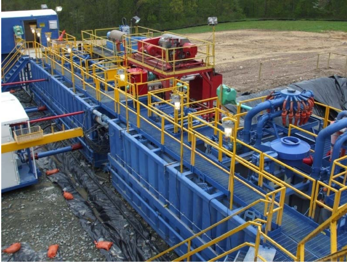
Photo 5.16 - Drilling rig mud system (blue tanks)
