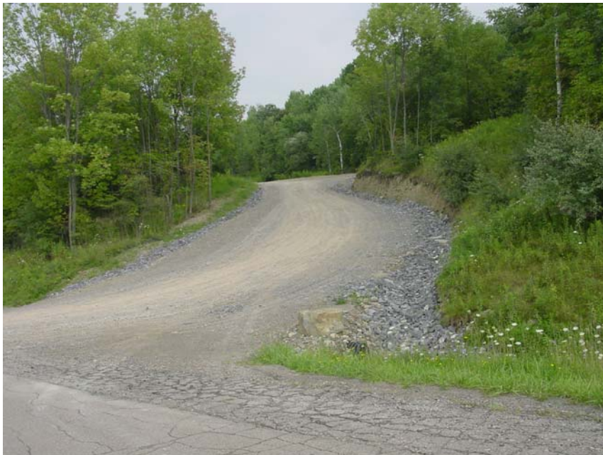
Photo 5.4 Access road and sedimentation controls, Moss 1, Corning, Steuben County NY. Photo taken during post-drilling phase. Access road at the curb is approximately 50 feet wide, narrowing to 33 feet wide between curb and access gate. The traveled part of the access road ranges between 13 and 19 feet wide. Access road length is approximately 1,100 feet long. Source: NYS DEC 2004.
