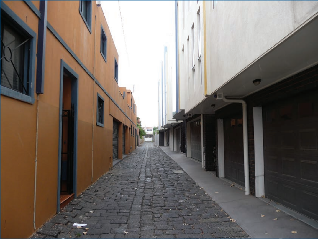
Hard surfaces cover the alley of a new development in the Melbourne suburb of Brunswick.
