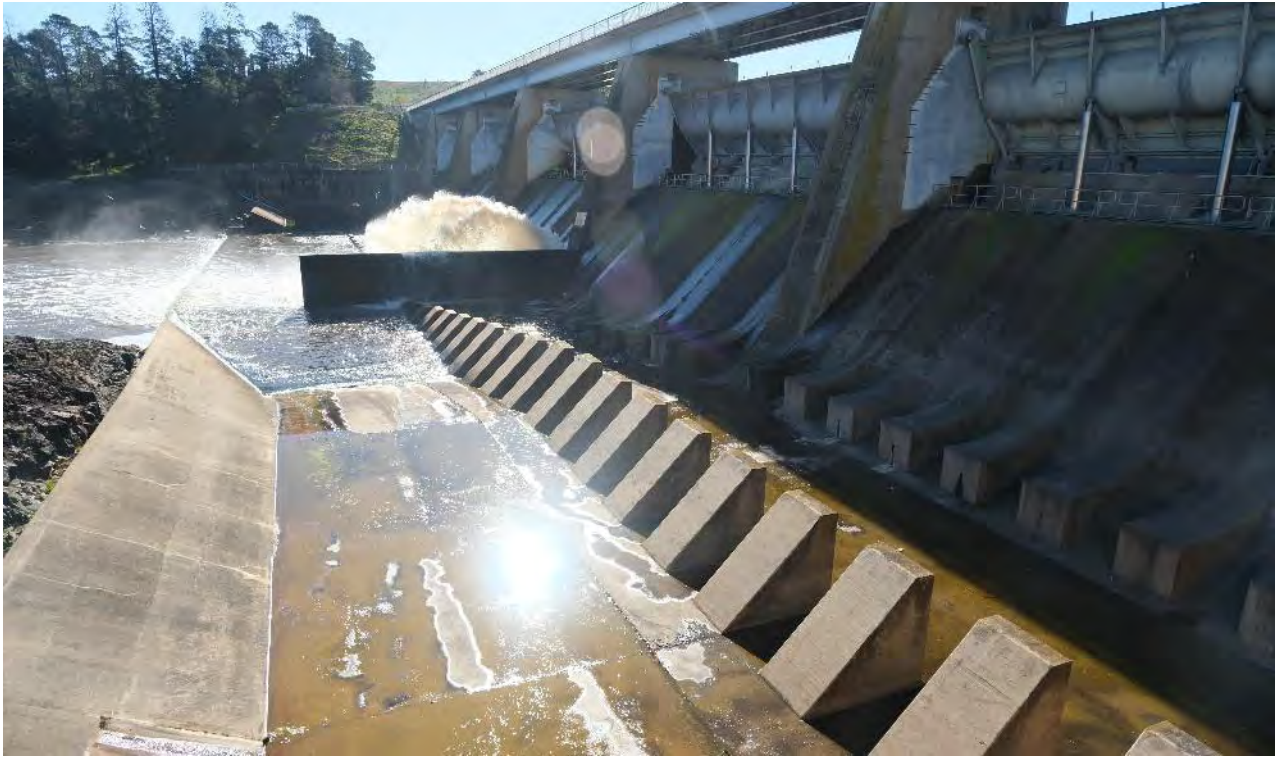
Photo B- 2.3 – -View of Chute blocks, apron and baffle piers
