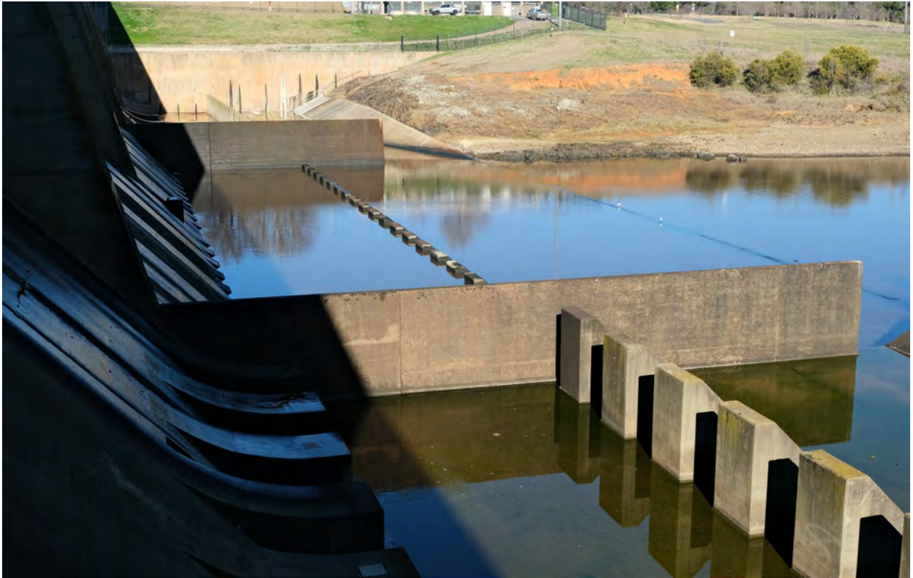
Photo B- 2.7 – Stilling Basin looking towards left side
