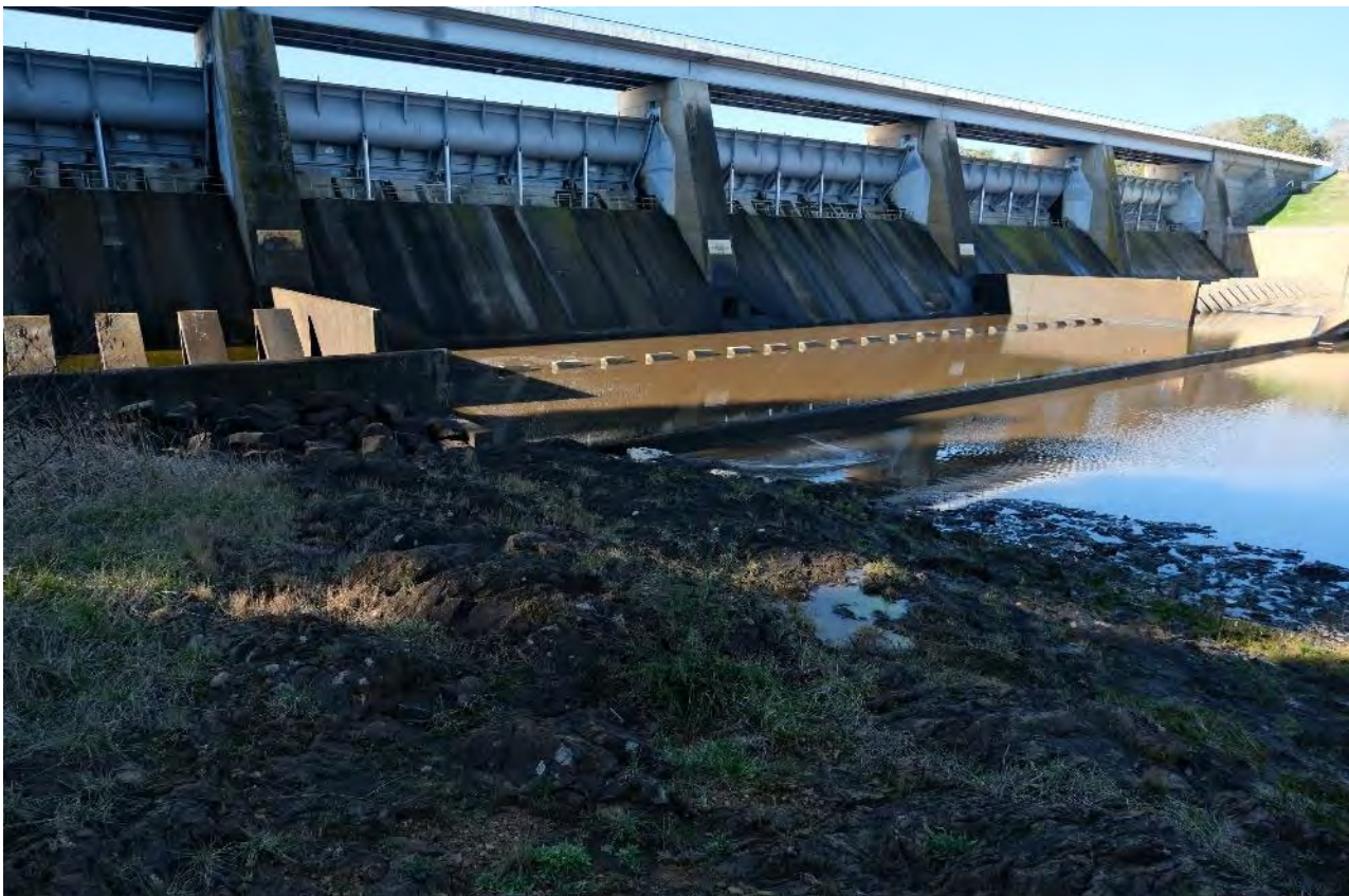
Photo B- 2.2 – -Photo of Overflow Section
