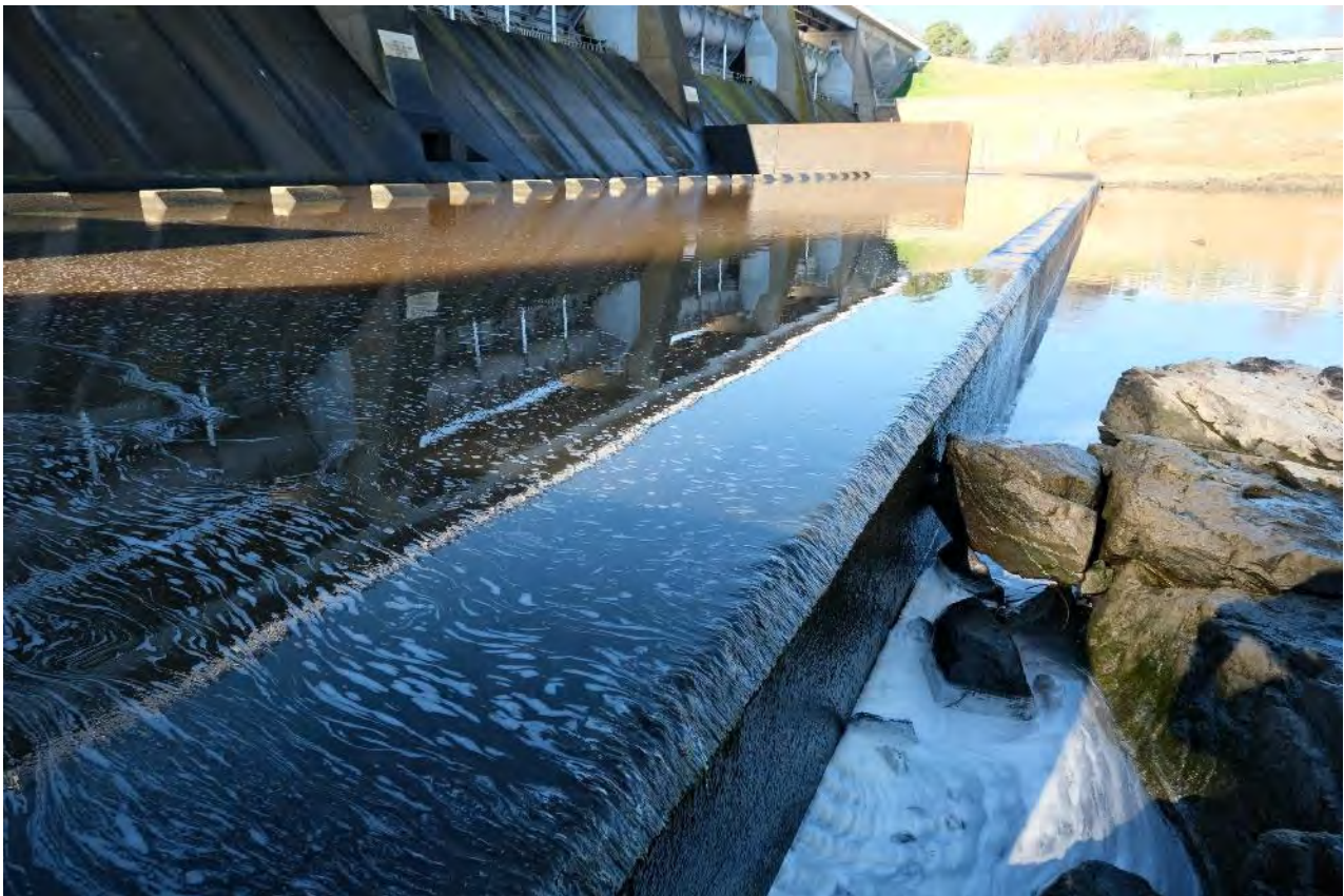
Photo B- 2.22 – Looking left along end sill
