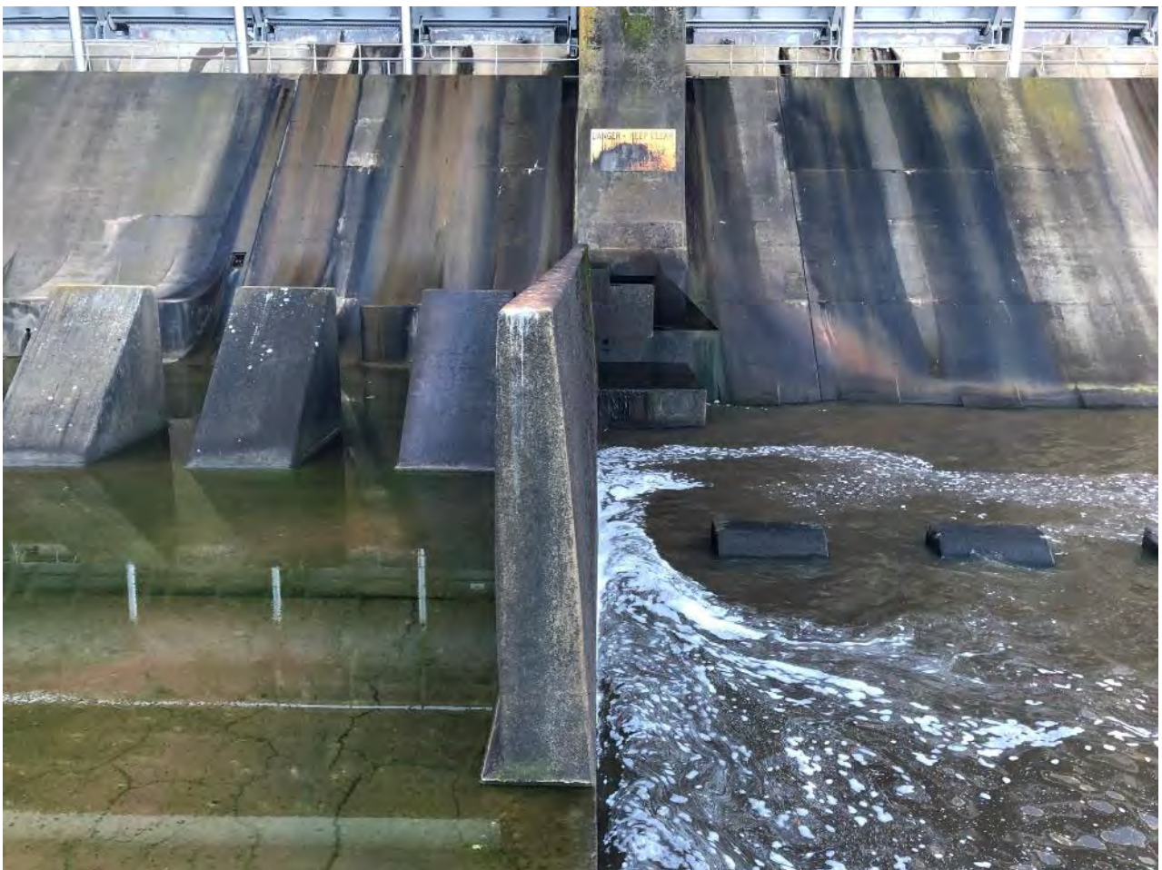
Photo B- 3.2 – Sluice Outlet
