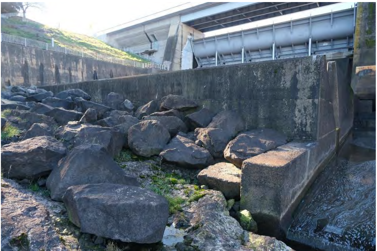
Photo B- 2.20 – Downstream end of Bay 1
