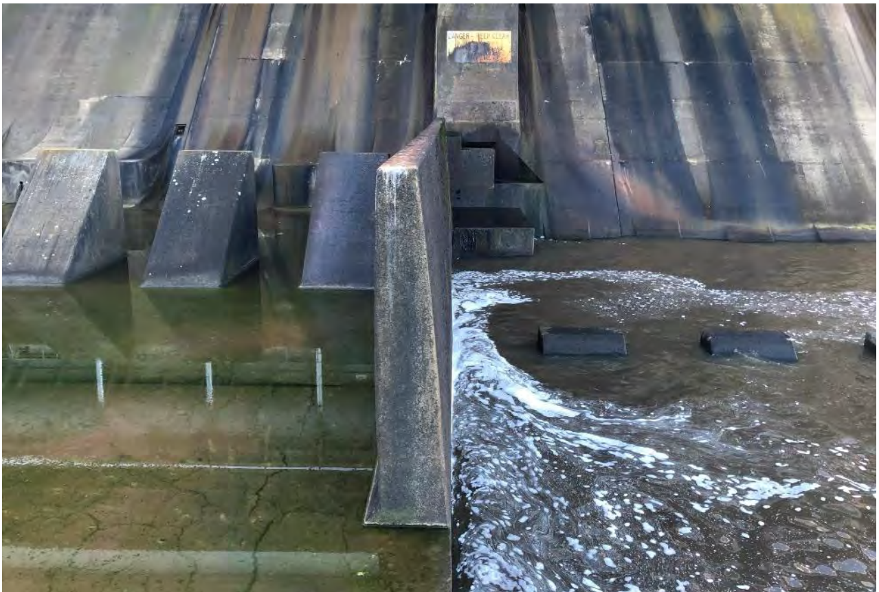
Photo B- 2.10 – Internal Splitter Wall in Stilling Basin
