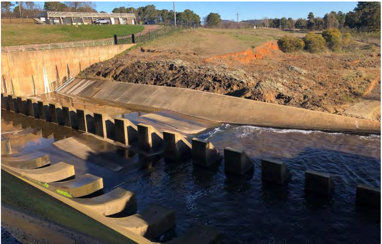
Photo B- 2.6 – Stilling Basin looking downstream and left
