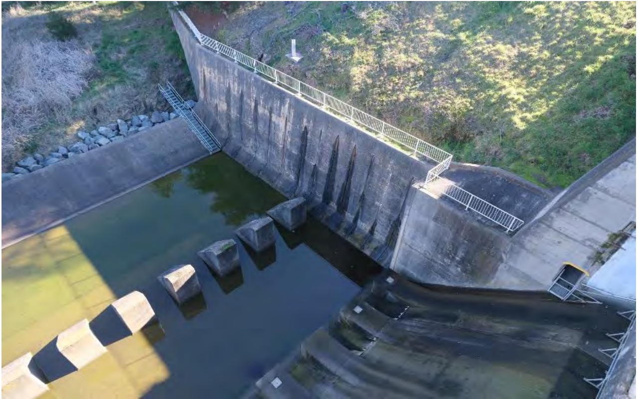
Photo B- 2.15 – Right downstream spillway training wall
