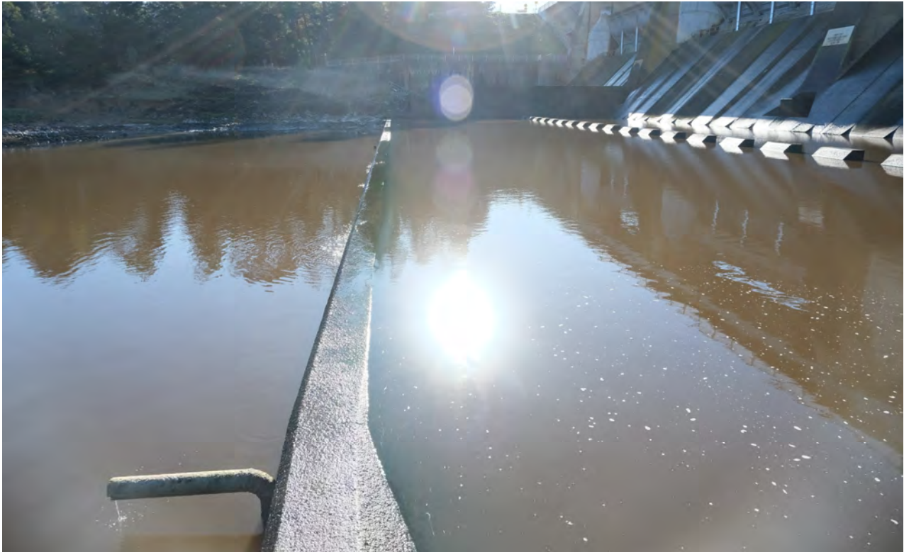
Photo B- 2.21 – Looking along End Sill
