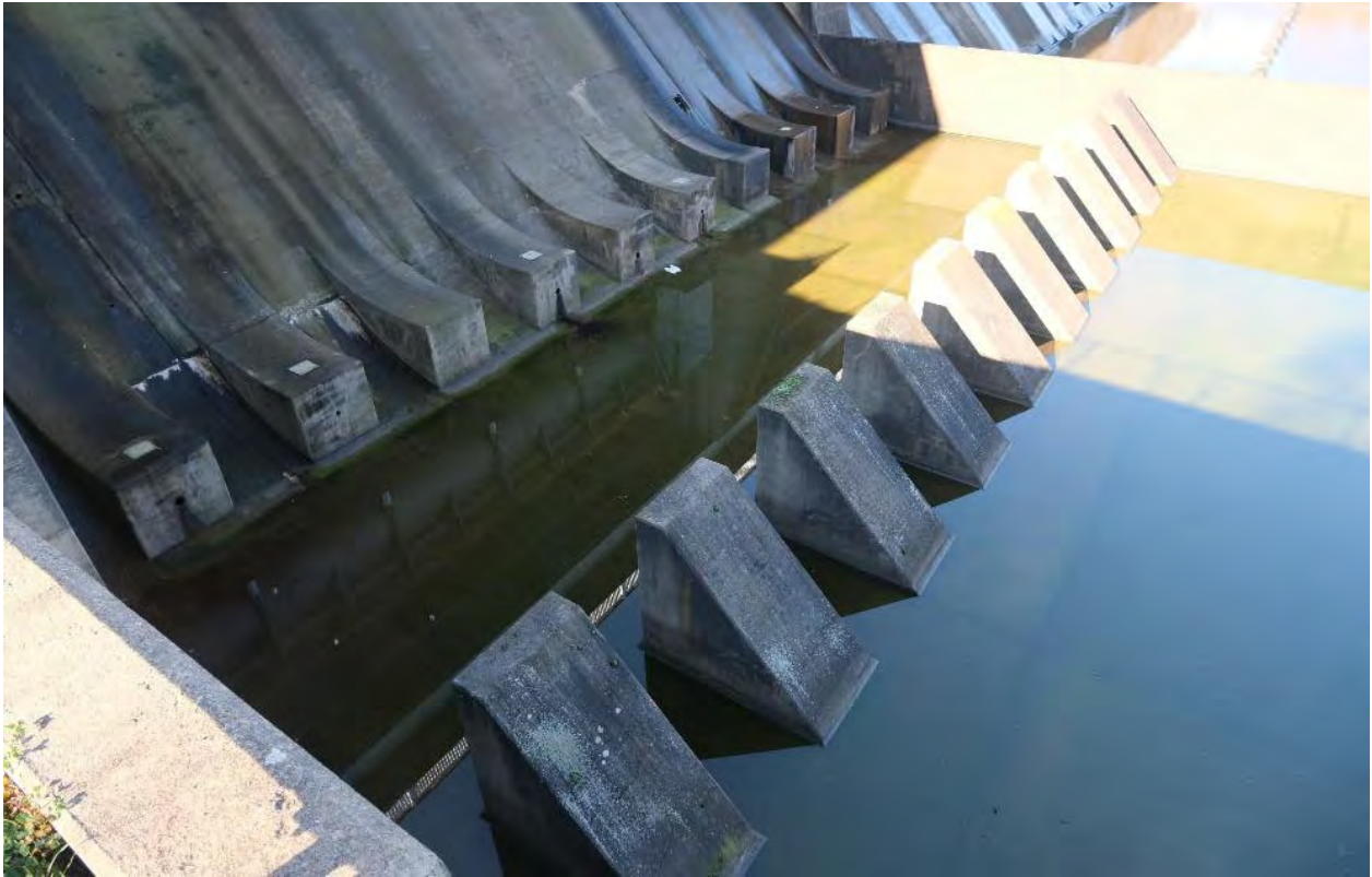
Photo B- 2.9 – Stilling Basin looking towards chute blocks and baffles
