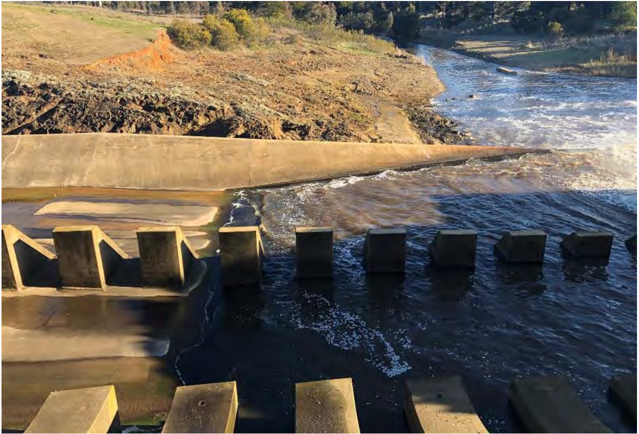
Photo B- 2.5 – Stilling Basin looking towards River
