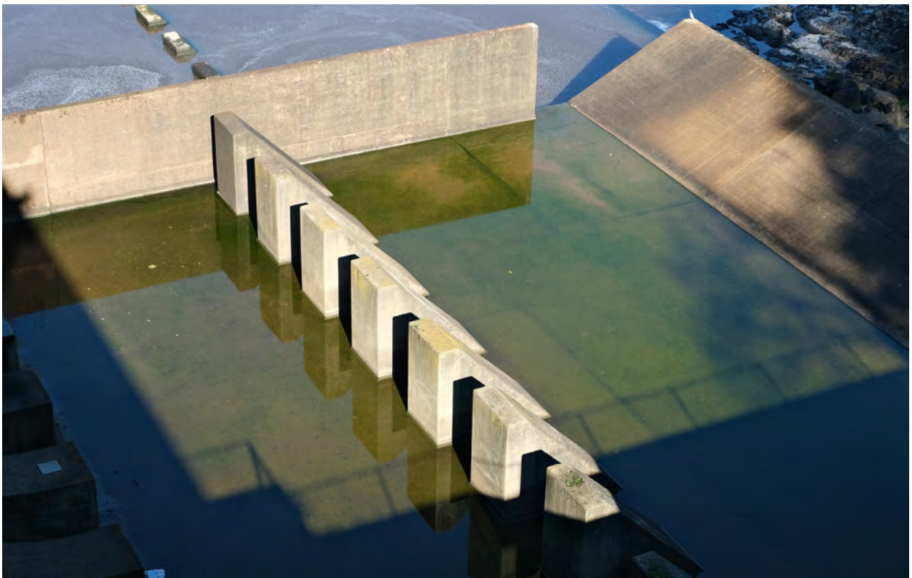
Photo B- 2.8 – Stilling Basin looking downstream to Bay 1
