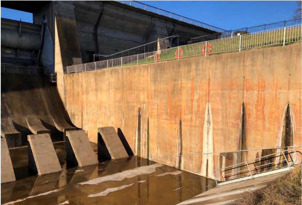
Photo B- 2.13 – Left downstream spillway training wall
