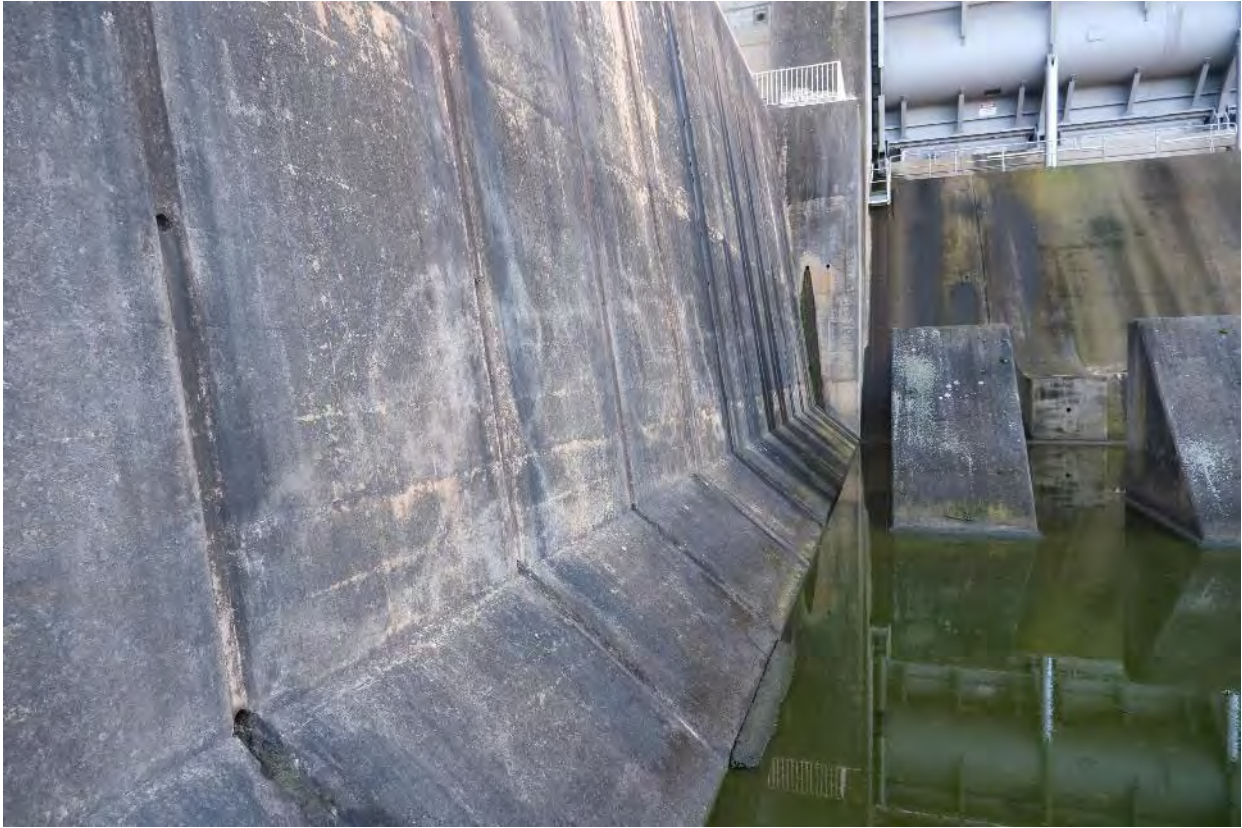
Photo B- 2.17 – Right downstream spillway training wall
