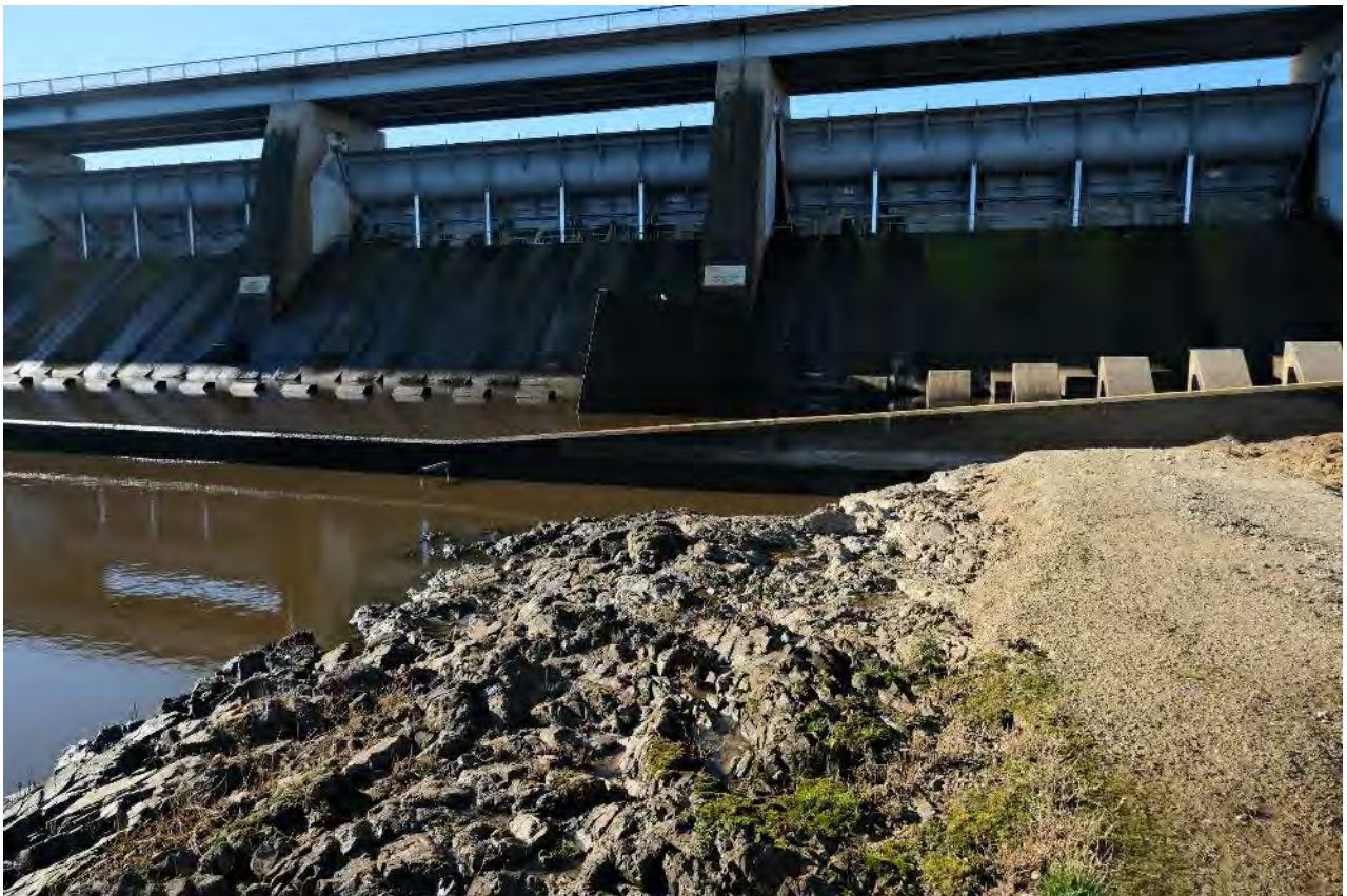
Photo B- 2.12 – Internal Splitter Wall in Stilling Basin
