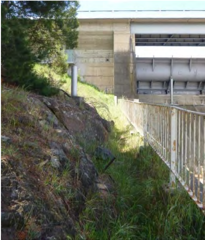
Photo B- 2.19 – Right downstream spillway training wall from Top
