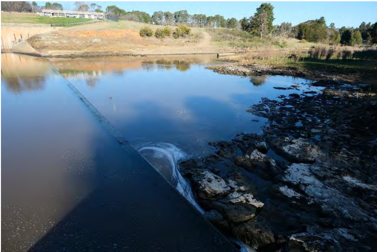
Photo B- 1.4 – View of area downstream from right abutment
