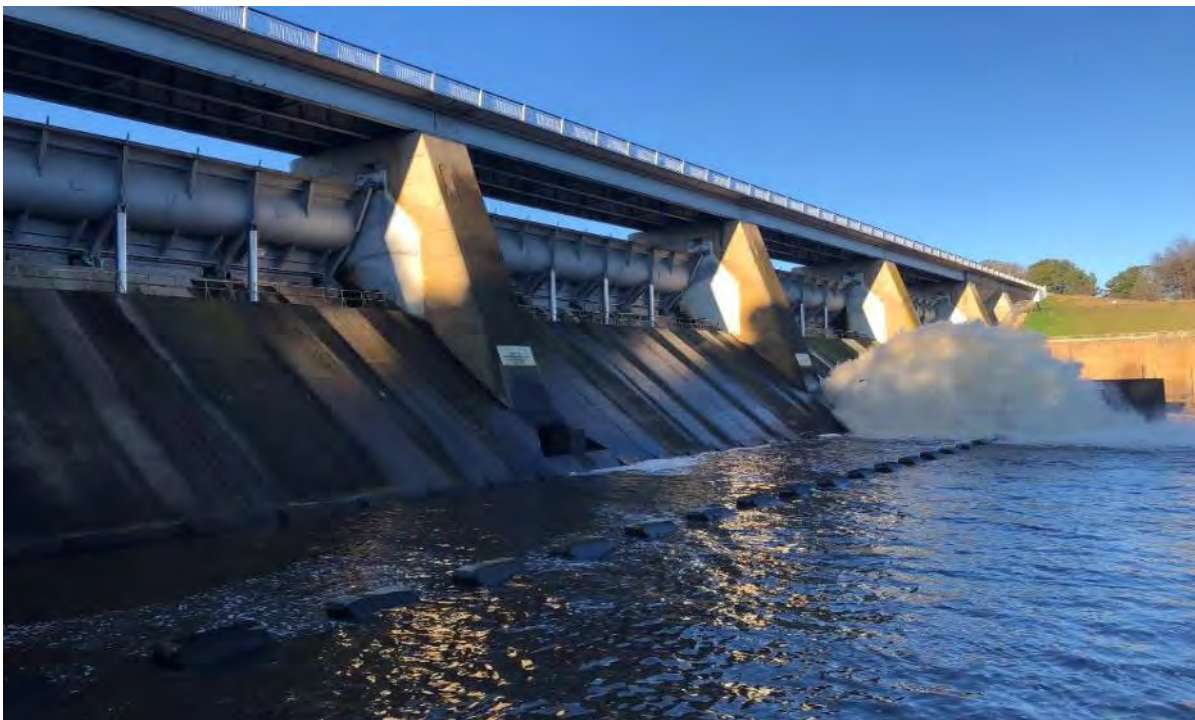
Photo B- 3.4 – Sluice Outlet
