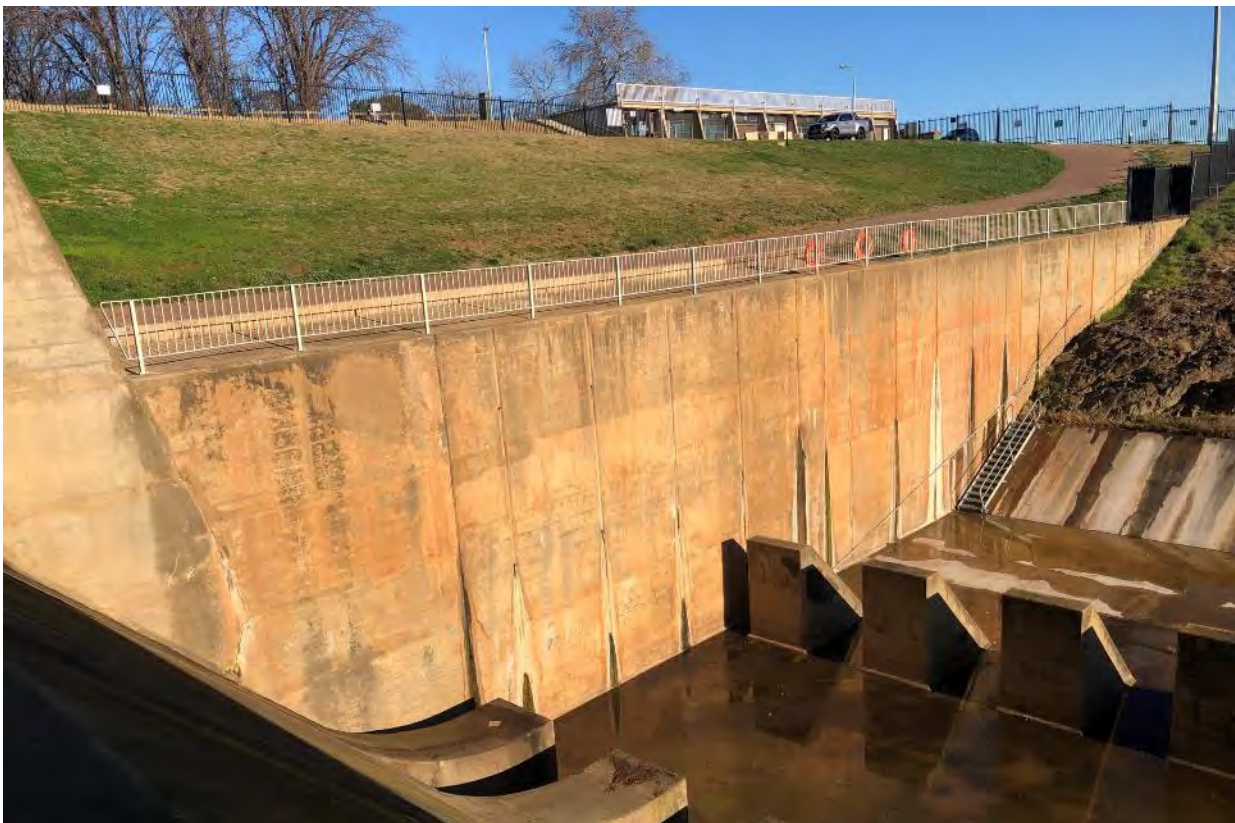
Photo B- 2.14 – Left Spillway Training Wall
