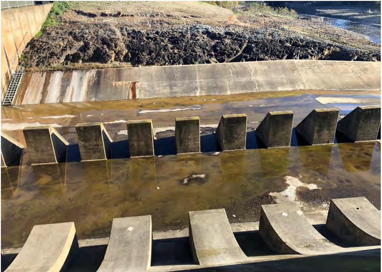
Photo B- 2.4 – View of Stilling Basin looking downstream (minor erosion downstream)
