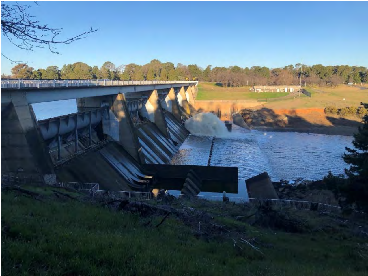
Photo B- 1.2 – Scrivener Dam looking towards left abutment
