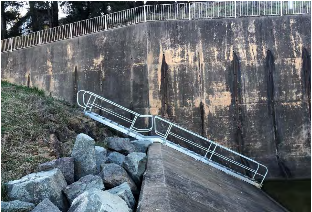
Photo B- 2.16 – Right Spillway Training Wall
