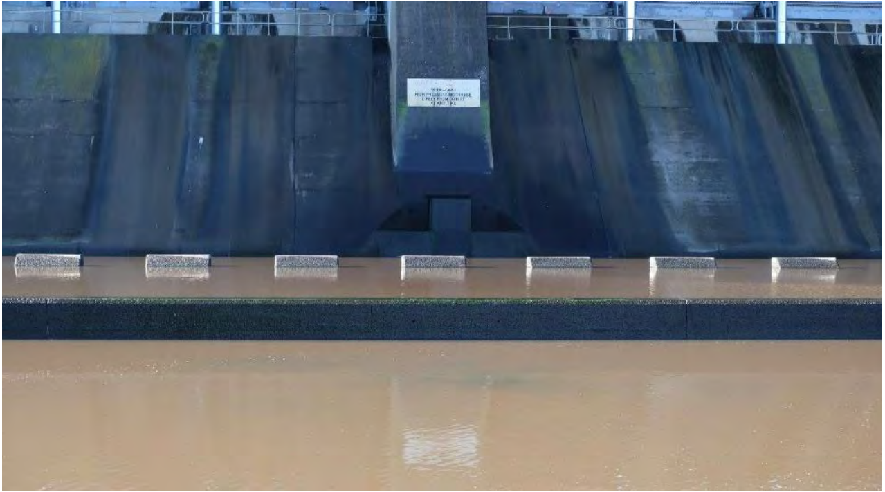
Photo B- 3.1 – Sluice Outlet Chute Block
