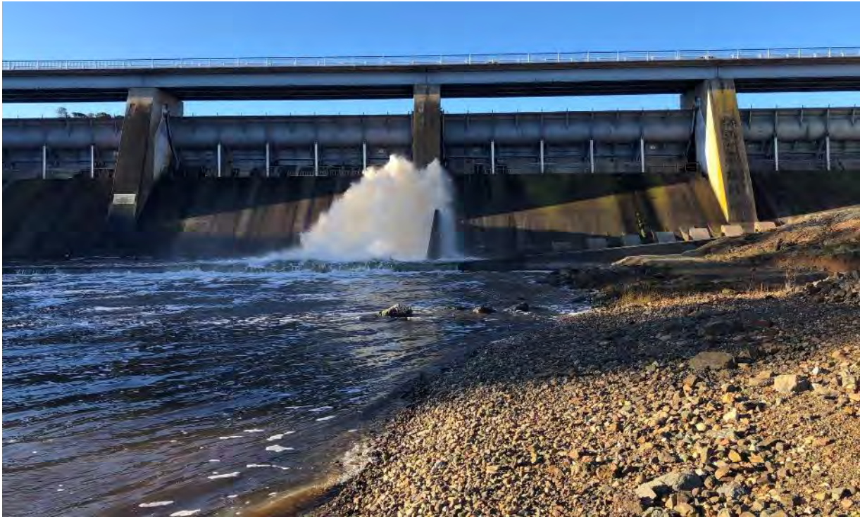
Photo B- 2.1 – Photo of Overflow Section
