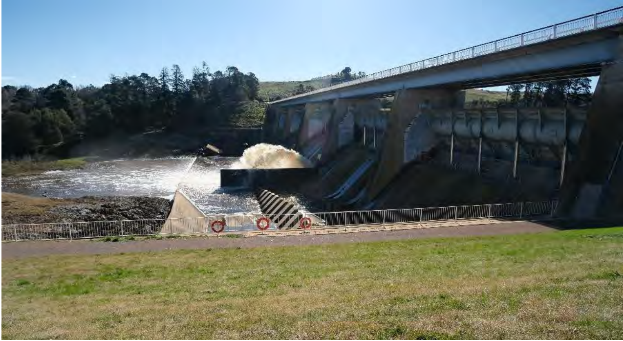
Photo B- 1.1 – View of Scrivener Dam from downstream
