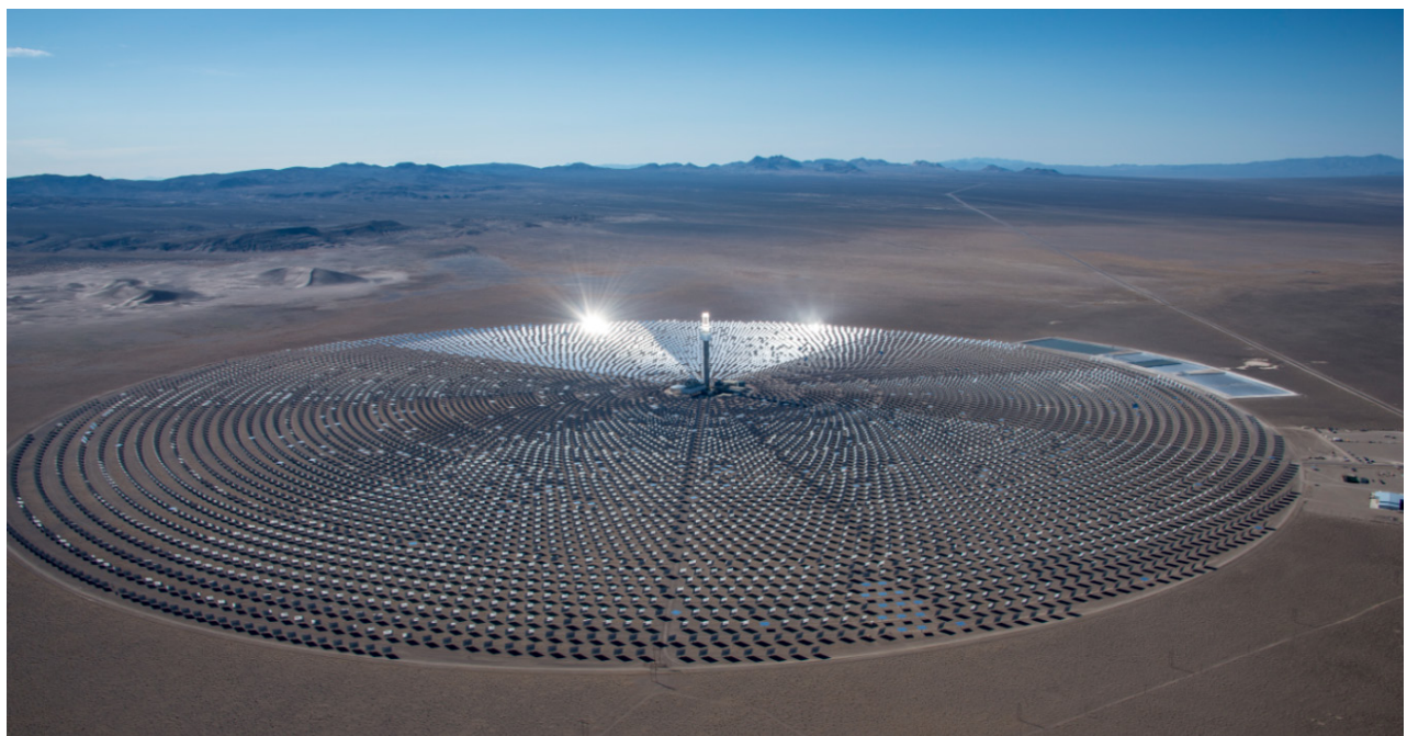
Crescent Dunes Solar Energy Project, Nevada, USA. 110MW with 10 hours of full load storage (1,100MWh)
