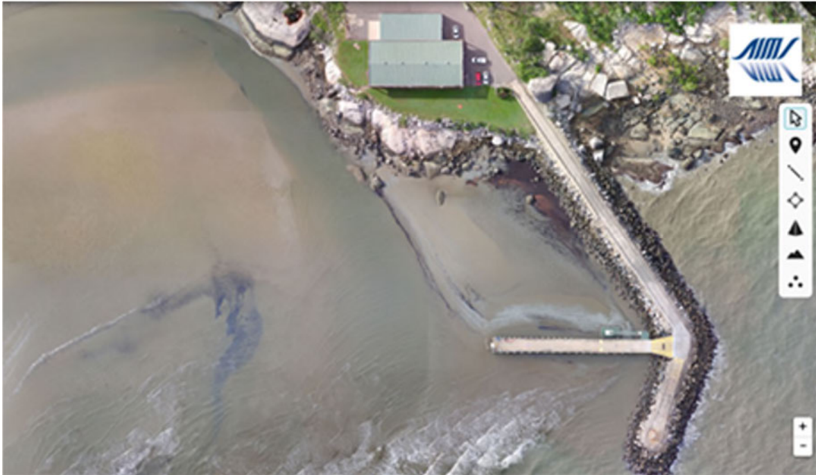
Figure 3: Aerial photo of AIMS' harbour showing the impact of sedimentation (2021). The wharf is now unusable, even at high tide.
