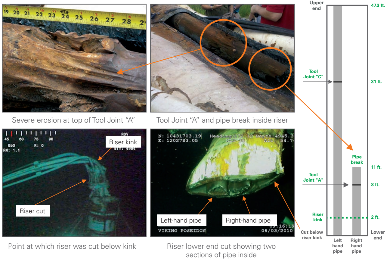
Figure 14. Retrieved Riser Kink Section and Its Contents.
