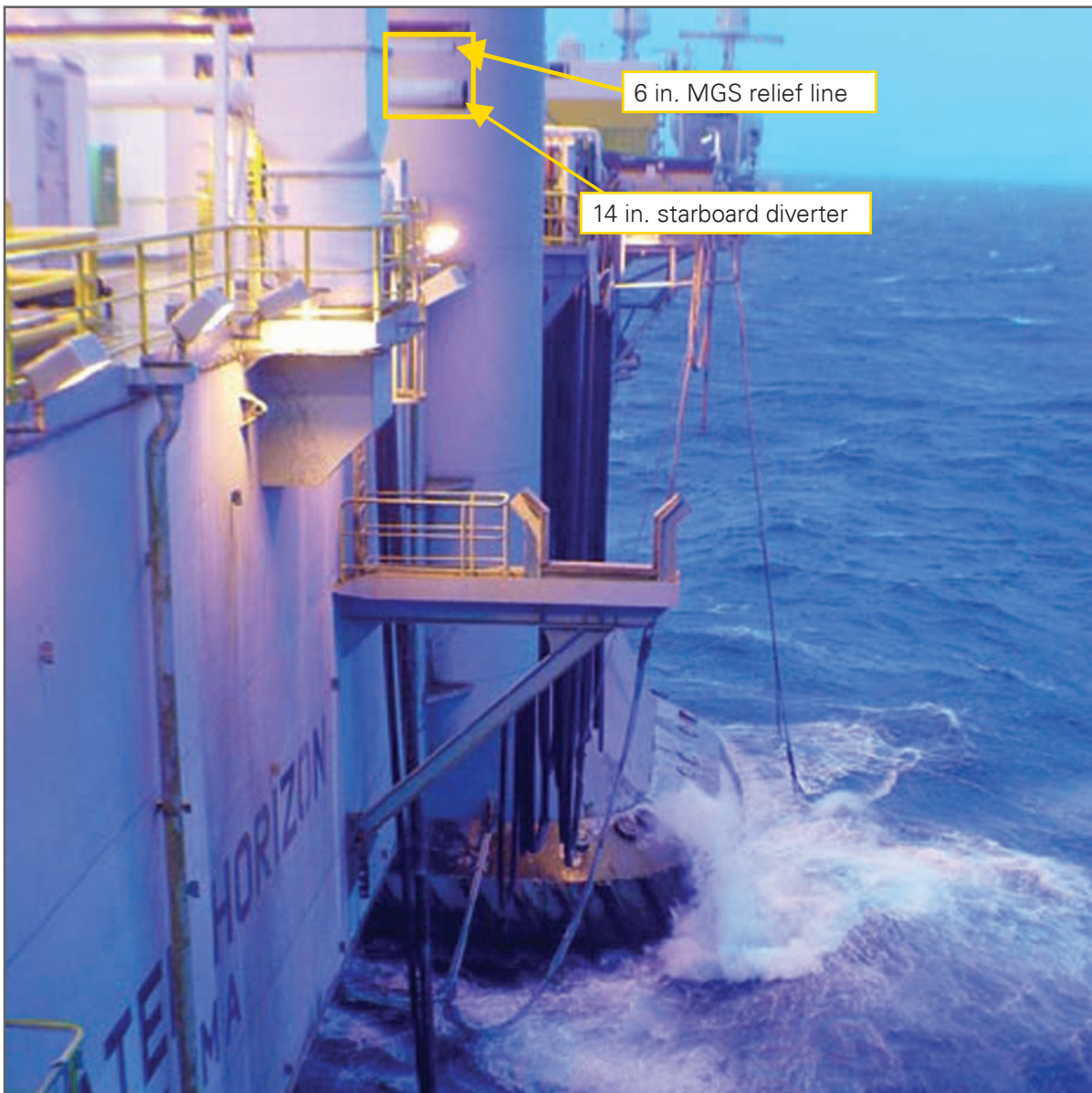
Figure 6. Photograph of Starboard Overboard Lines.
