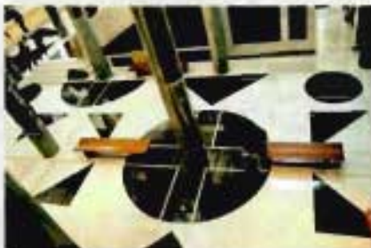
Sadubin benches being installed
