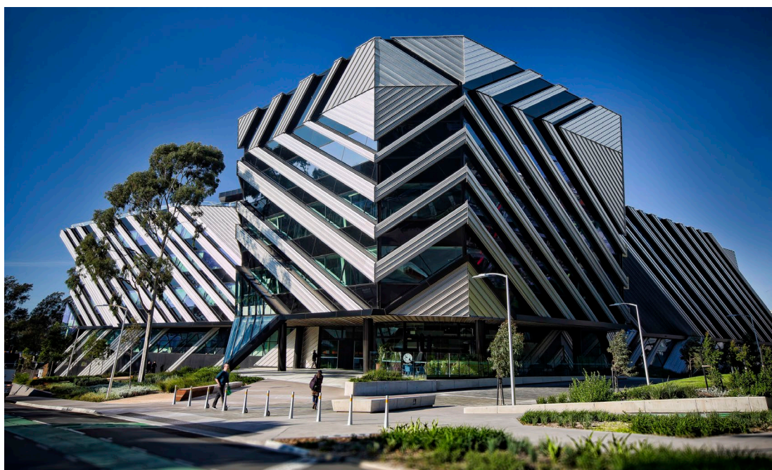
New Horizons building, Monash University, Clayton campus
