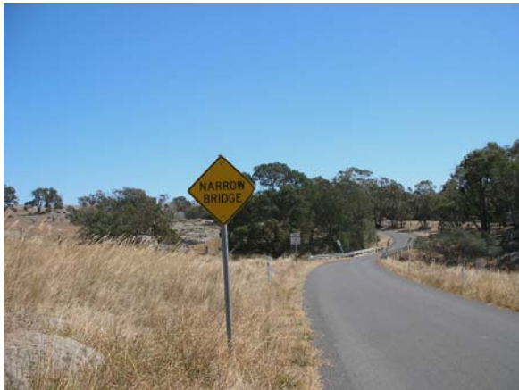
Narrow road and bridge one of only two access roads
