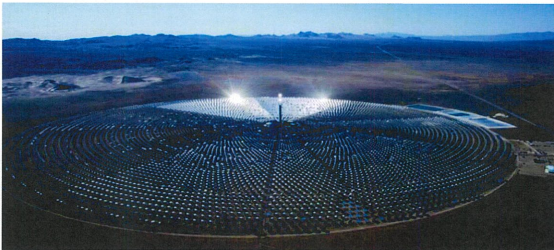
Crescent Dunes Solar Energy Project, Nevada, USA. 110 MW with 10 hours (1,100 MWh) full load storage (SolarReserve)
