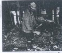
Destroyed: Toodyay is rebuilding after the devastating blaze in December.
