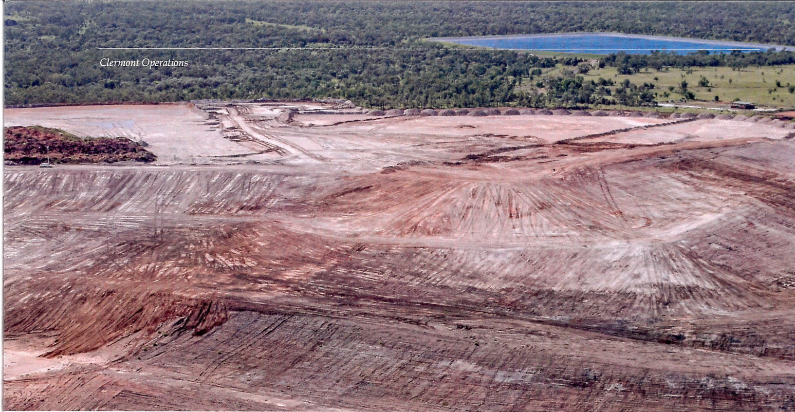
Shaping work (above) on Clermont's Northern West Rock Dump and rehabilitation progress (below).
