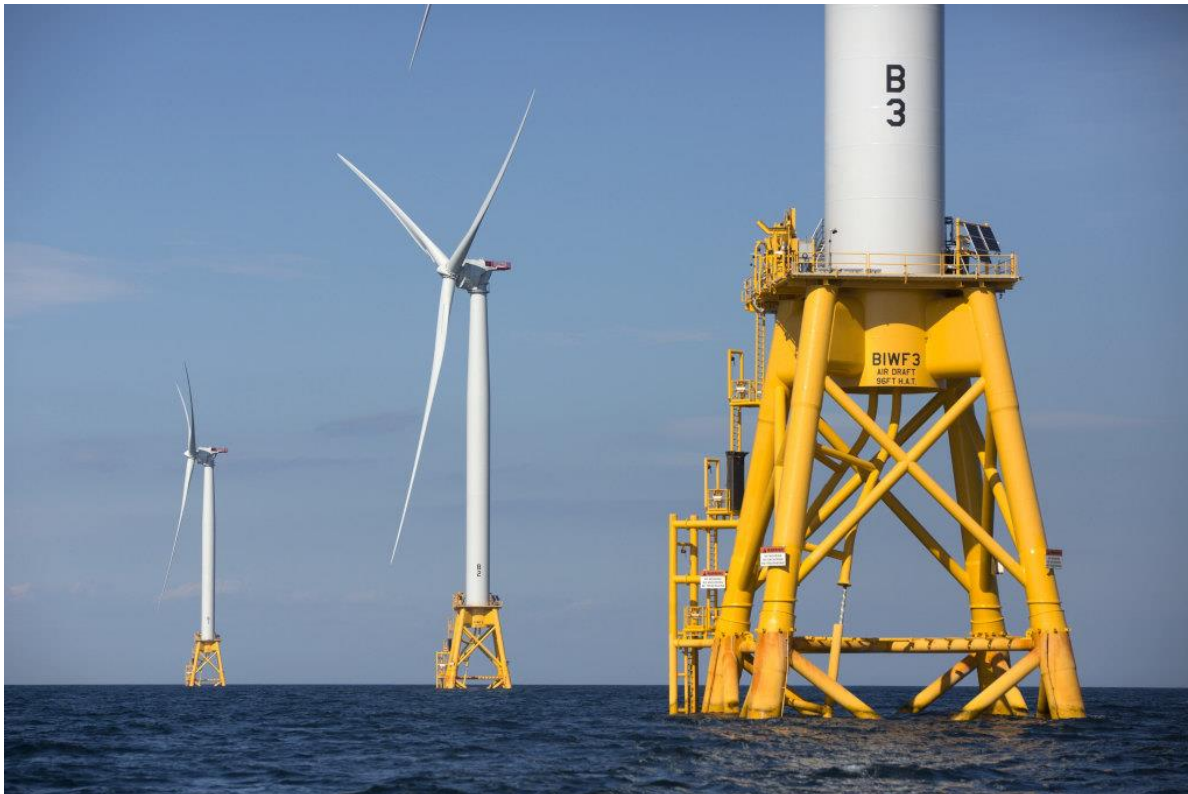
Figure 2. An example of a desirable windfarm design (multiple pole platforms) which would have a much greater fisheries enhancement effect compared to Figure 1, due to greatly increased internal void area and abundant horizontal cover. These installations are effectively true artificial reefs.
