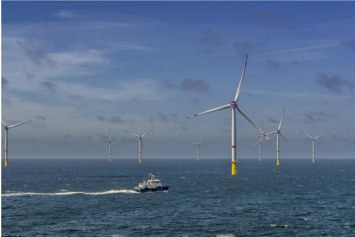
Figure 1. An example of a windfarm design (single poles) which provides minimal value for enhancing fisheries production, due to reduced surface area and lack of horizontal cover.
