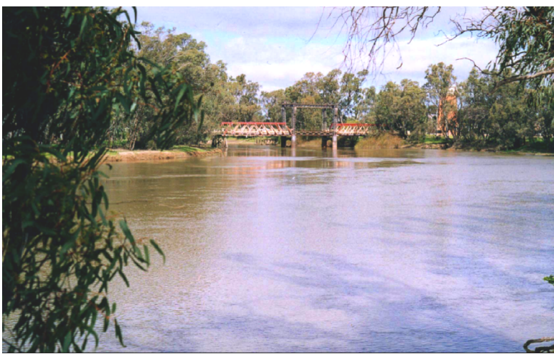
Photo 1: Swan Hill Murray River bridge and water tower in the huge 2003 drought.
