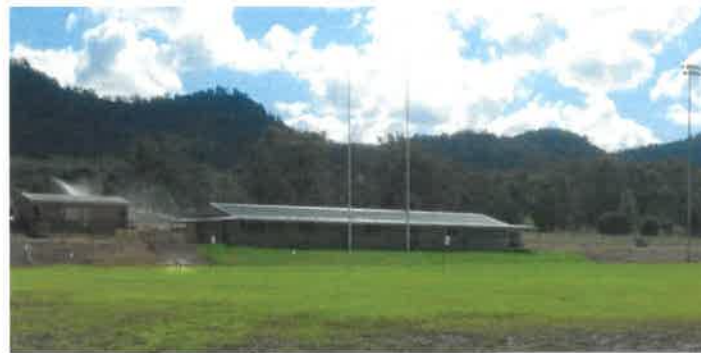
Denman Recreation Centre $3.4 million through Mangoola VPA
