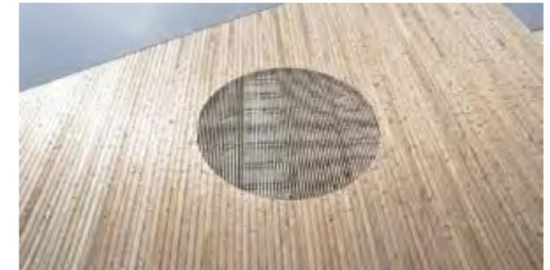
Steel structure with angulated timber slats
