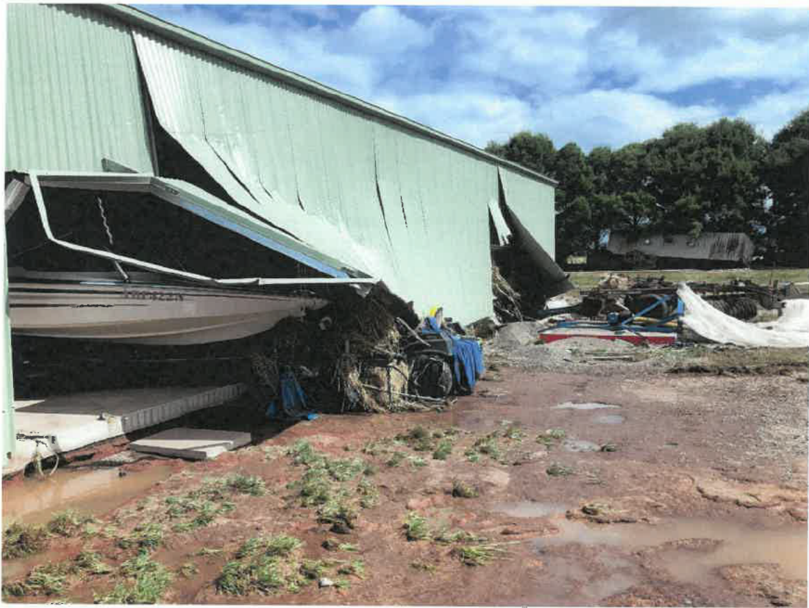
Photo 9: image of another shed on the subject property. This photo shows the western side of the shed blown out and a boat that was originally parked pointing to the south, now pointing to the south west. Had that impact this property only originated from the north, it would have flowed in parallel with the sheds and pushed all that was inside out the southern end. Furthermore, the right-hand side of this image shows a shipping container that was originally placed east to west, it is now clearly on an angle (source: personal image taken on subject property).
