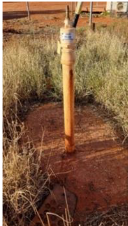
2. Fire hydrant missing connector
