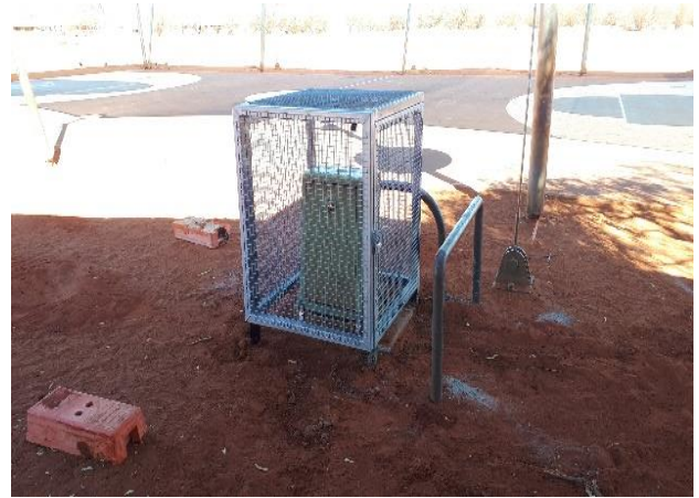
4. Power pillar protection measure
