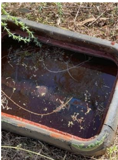
3. Potable water pit with leak
