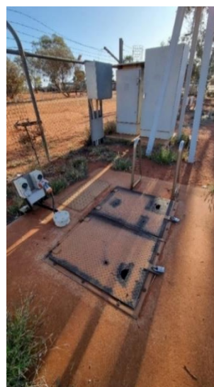
6. Ageing sewer pump station
