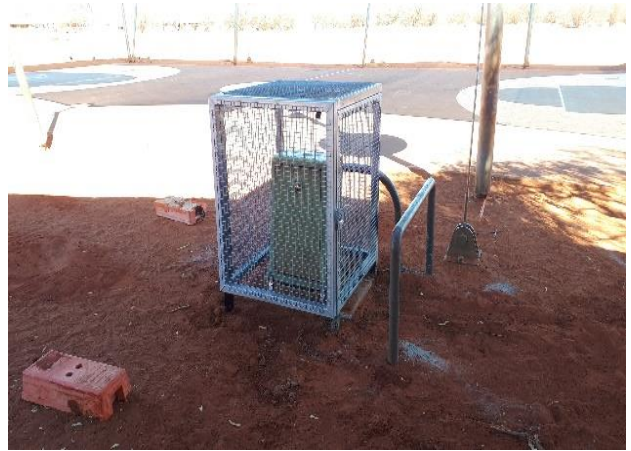
4. Power pillar protection measure
