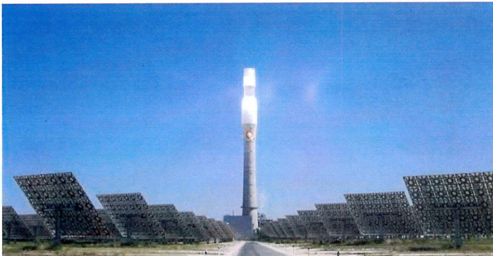
Figure 5: Concentrating Solar Thermal power station.
