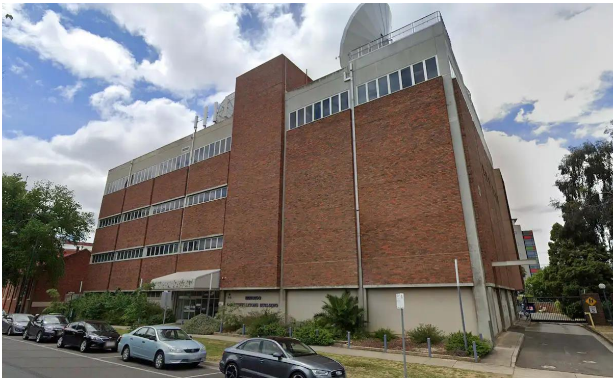
Figure 5. An exchange building in Bendigo, Victoria. Google maps, CC BY-SA (Gregory, 2023c)
