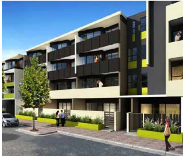
Two units are located on the ground floor with direct access from street level, artists impression, Hunter Demonstration Project.
