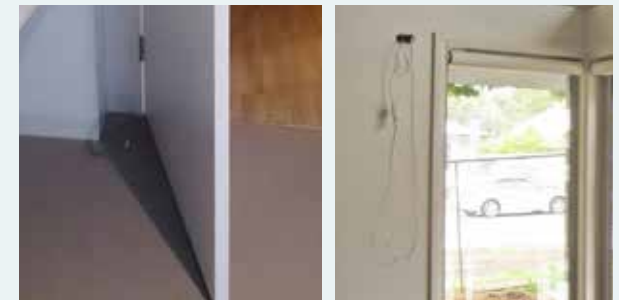
Slimline wall corner guards and timber-look vinyl flooring, Abbotsford (left) and pre-wiring for future blind automation prior to install of coverplates, TAC RIPL Housing (right).
