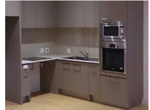
Removed underbench cabinetry post tenant modifications, Abbotsford
