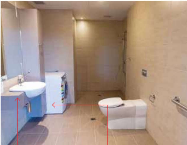
person with small stature cannot see themselves in the mirror and basin height is fixed
