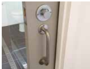
D-pull handle, required to achieve platinum level.
