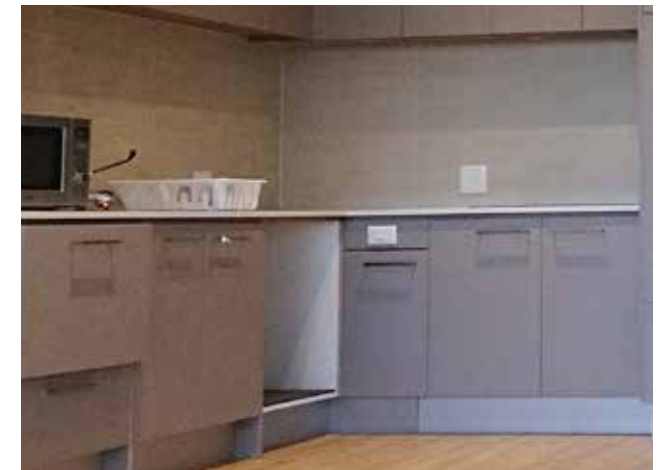
Post individual modifications, corner underbench cupboard removed to allow use of the cooktop by a person with reclined posture.
