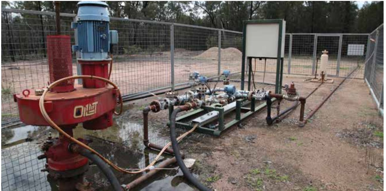
Figure 4.1: Decommissioned coal seam gas well, Pilliga Forest
