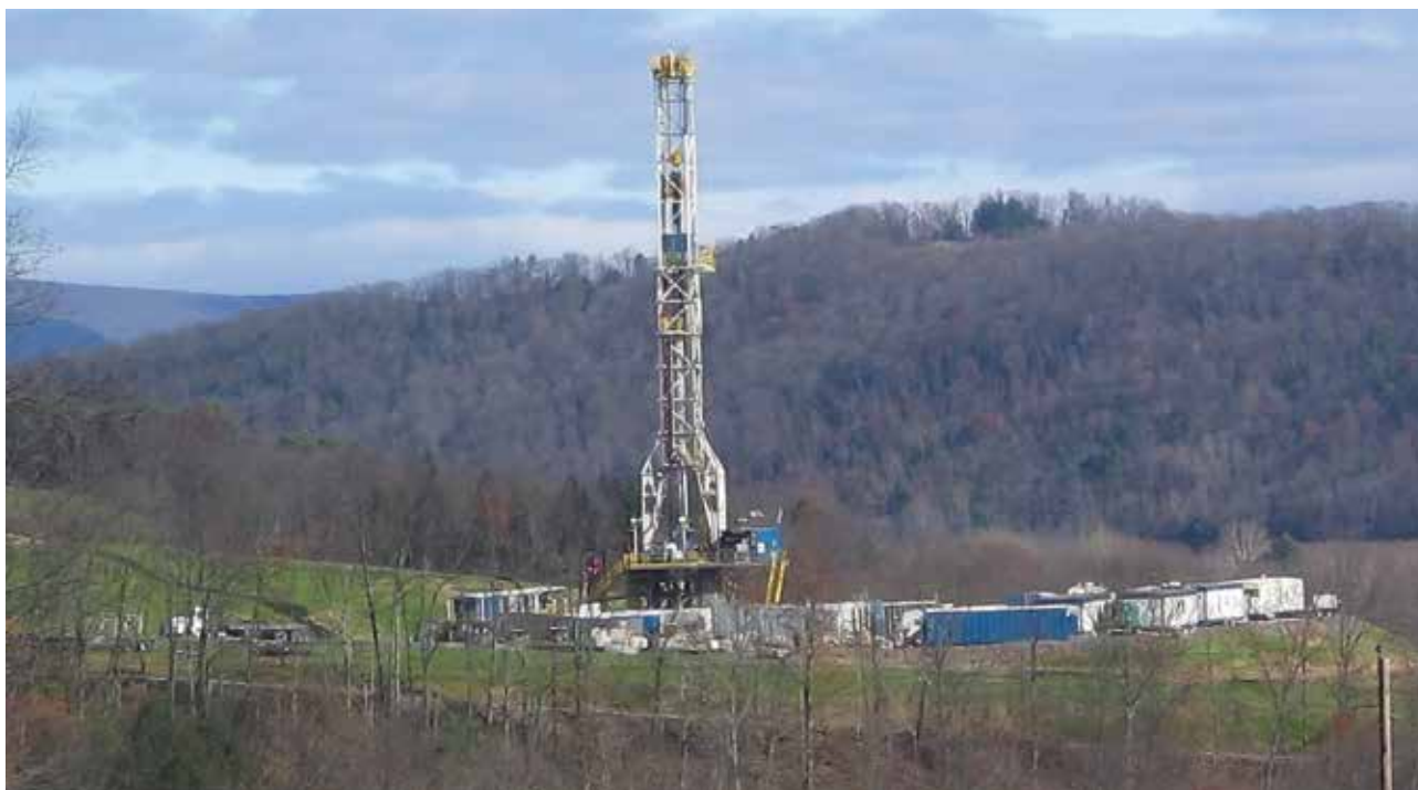
Figure 2.2: Tower for drilling horizontally into the Marcellus Shale Formation for natural gas in Lycoming County, Pennsylvania, USA
