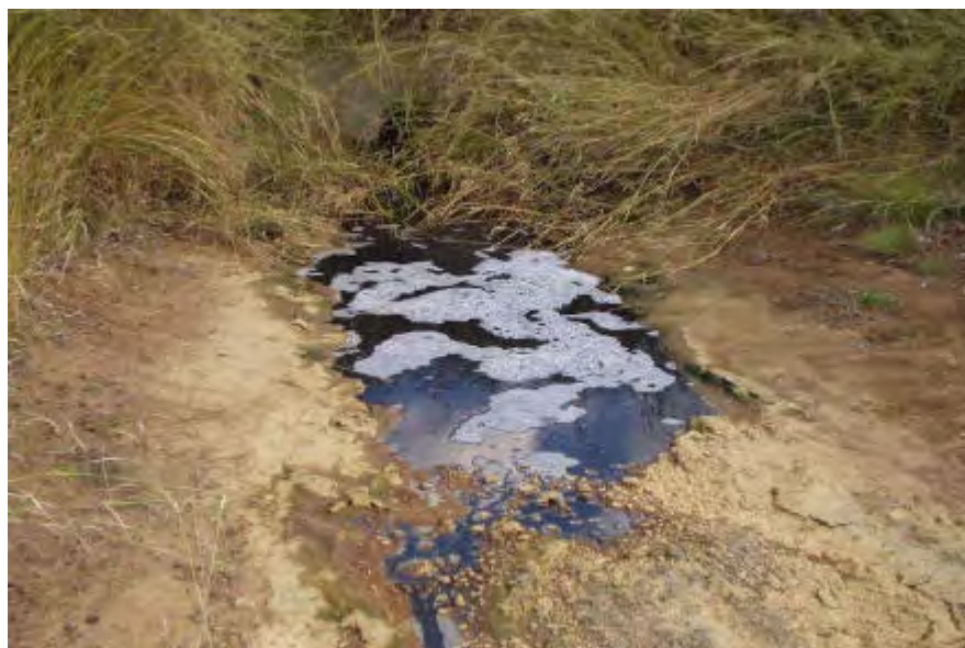
Figure 4.6. Foam waste-water leaking from a collection pit drain within Defence land (RAAF Amberley).
