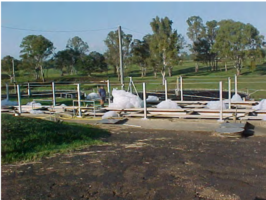
Figure 3.2. Excess foaming caused by AFFF waste at RAAF Amberley water treatment facility. (The excess foaming is not due to any fault of the sewage treatment plant operator.)
