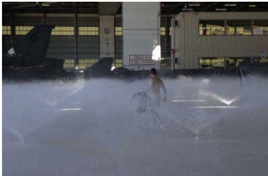
Figure 2.4 Current practices for managing exposure to AFFF by Defence leave a lot to be desired. Here foam samples are collected during a test, but without protective clothing.
