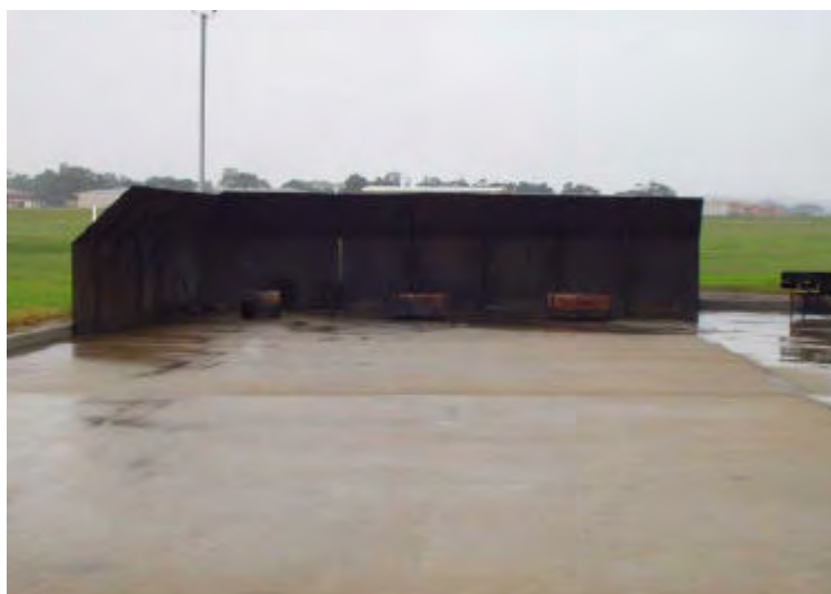
Figure 4.5. An example of a purpose built crash crew vehicle testing/fire training facility at a RAAF Williamtown.
