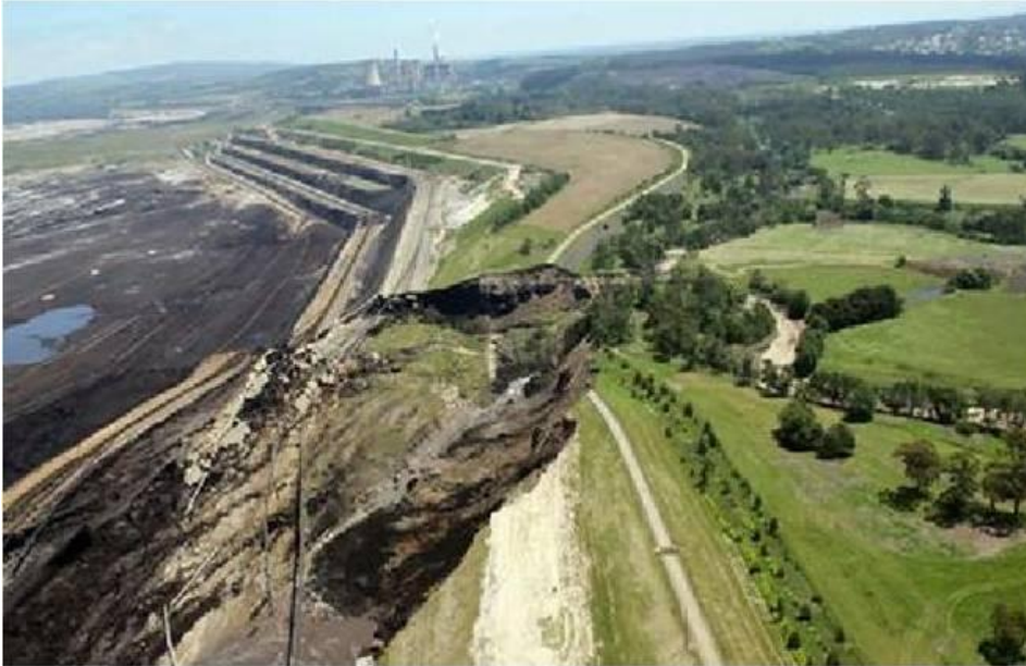
Figure 4: In 2007, the Latrobe River was lost into the Yallourn open cut coal mine following collapse of the mine wall. The Government Inquiry into the disaster identified slack and lapsed safety standards and found that mine consultants had lacked the skill to give competent advice 17
