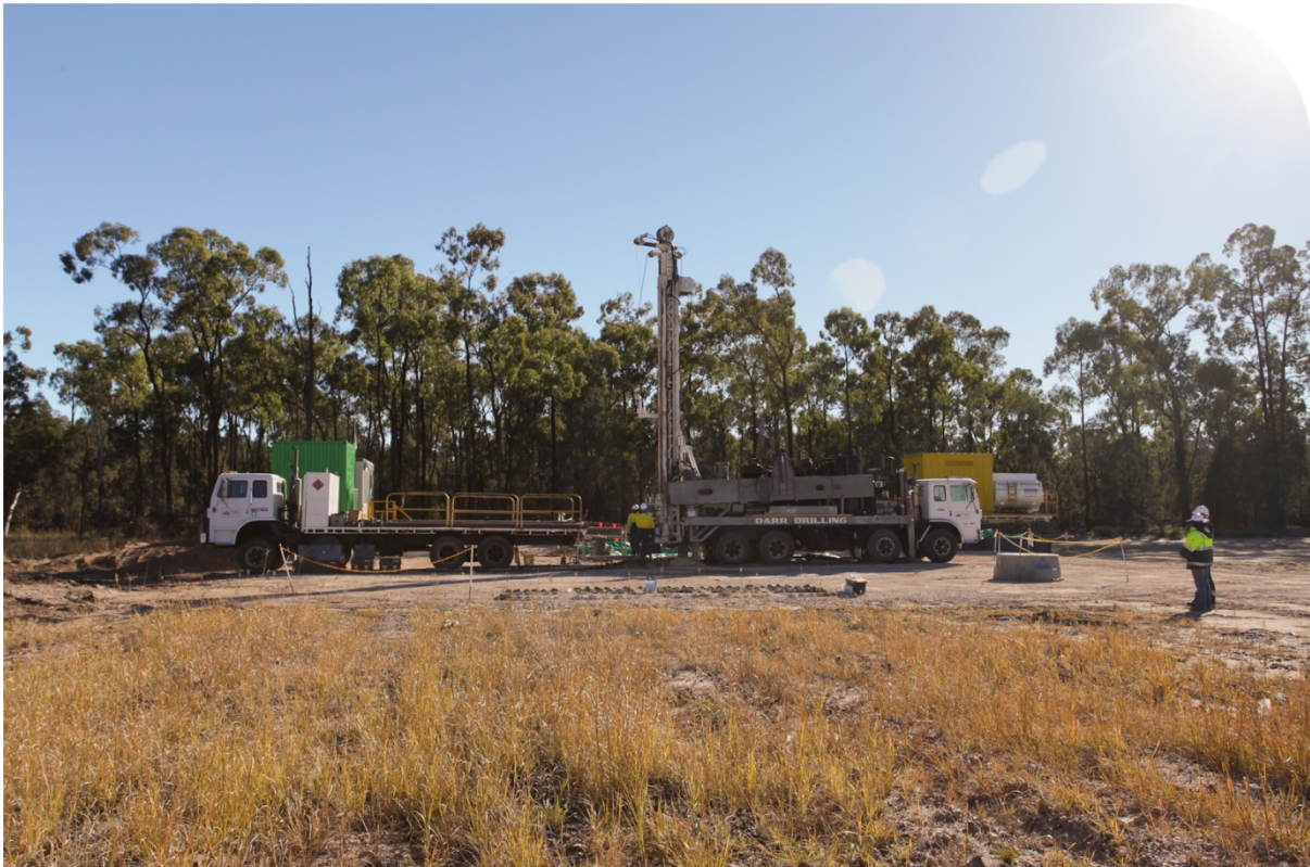
Installation of one of Australia Pacific LNG's many new monitoring bores
